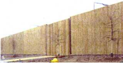
Parking area exterior fence/gate
