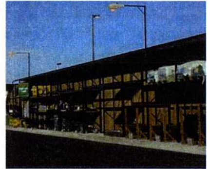
Pallet rack interior fence
