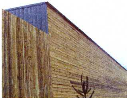
Pallet rack exterior fence at warehouse back wall siding
