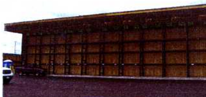
Warehouse front wall siding
