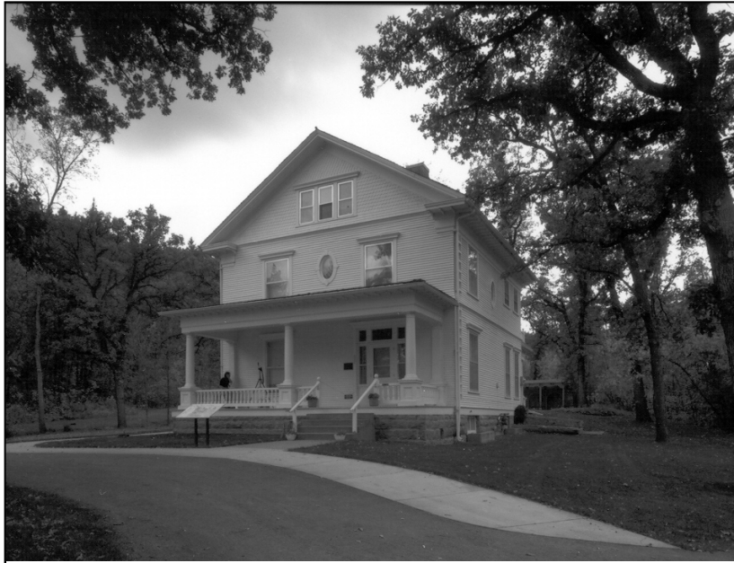
Figure 9 – The Superintendent residence at the DC Booth National Fish Hatchery was listed on the National Register of Historic Places as part of the Spearfish Fisheries Center historic district. The district is significant under Criterion A in the area of conservation, serving the Black Hills and upper plains regions as a principal fish rearing and management facility since 1898.
