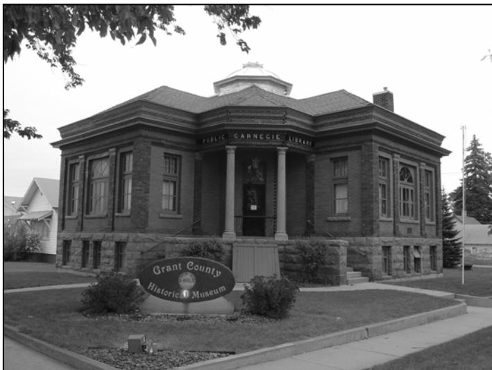
Figure 2 – Many quality-of-life activities are often housed in historic buildings. The former Milbank Carnegie Library is now home to the Grant County Historical Society museum.
