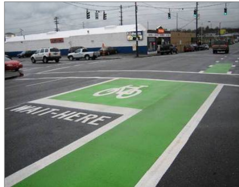
Figure 58. Bike boxes have been installed at several intersections in Portland, OR where right-turning motorists conflict with through bicyclists.
