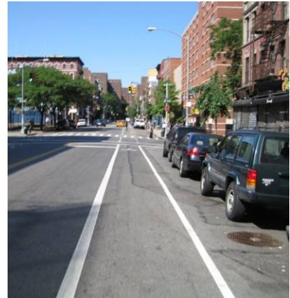
Bike lanes provide a travel lane for bicyclists that is separated from motor vehicle travel and parking lanes.
