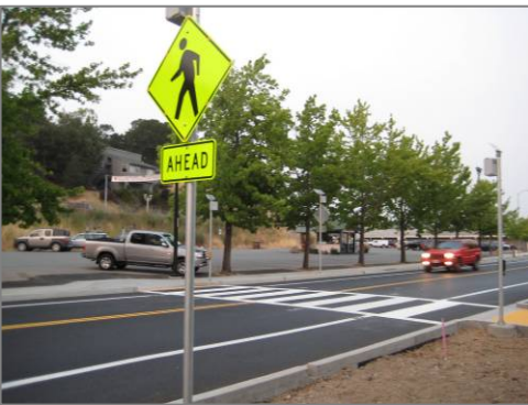
Figure 48. Example high-visibility crosswalk with fresh paint and a warning sign with flashing lights.
