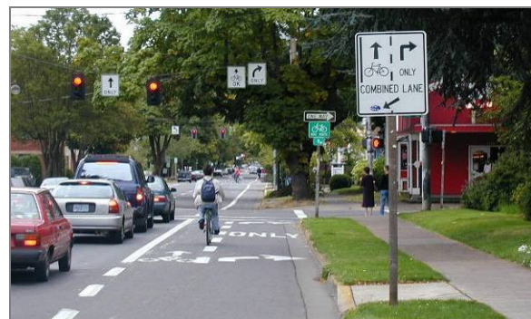
Shared bike-right turn lanes require warning signage as well as pavement markings
