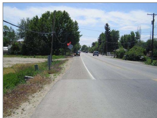
Shoulder bikeways are appropriate along wide rural roads where vehicles can avoid passing close to bicyclists.
