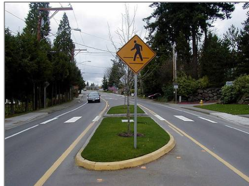
Figure 42. Pedestrian refuge island at mid-block crossing.
