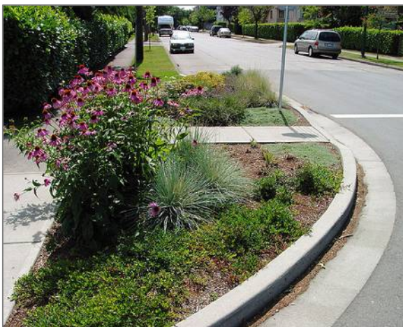
Figure 41. Planted curb extension in Portland, OR
