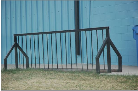
Figure 16. Bike racks provided at several schools do not support bicycles when they are locked.
