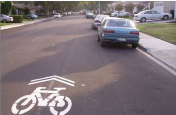
Figure 13. Shared lane marking treatments improve visibility of bicyclists on streets where bicyclists and automobiles share a travel lane.
