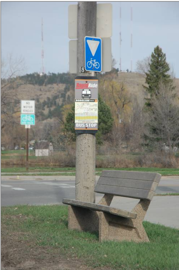
Figure 17. RapidRide bus stop with a bench but no concrete waiting pad between the street and sidewalk.
