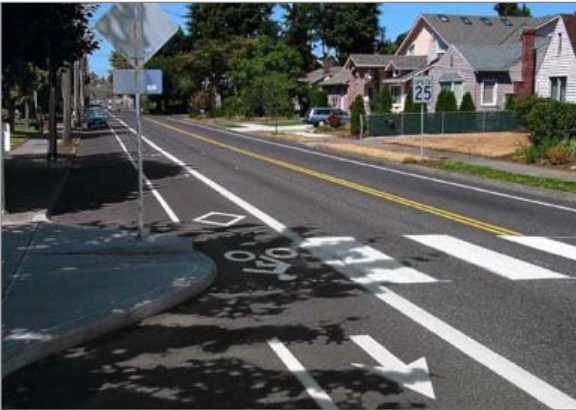
Figure 12. Designated bike lanes are designated with pavement markings and signs, and parking is prohibited.
