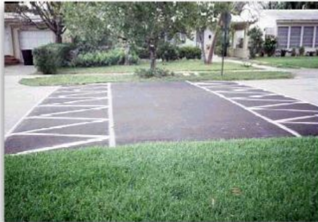
Illustration of a Speed Table
