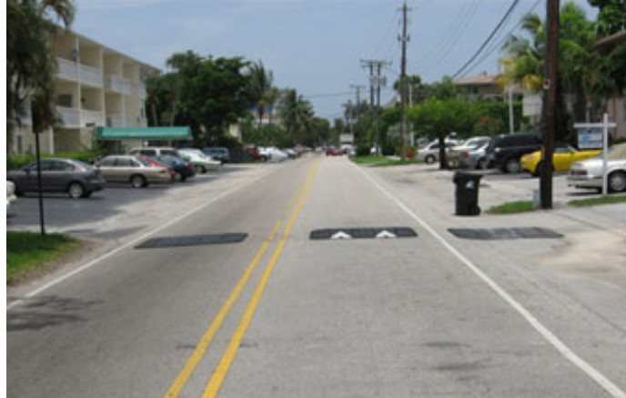
Illustration of a Speed Cushion
