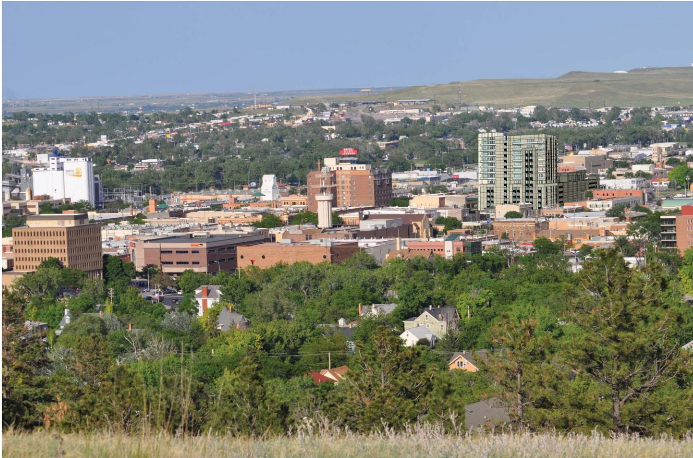
Skyline View from South-West of Project Site
