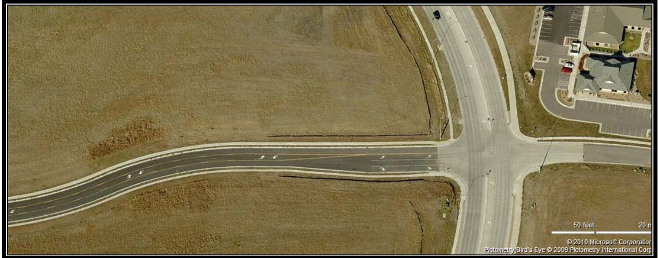
Figure 3: 5 th Street and Stumer Road Intersection
