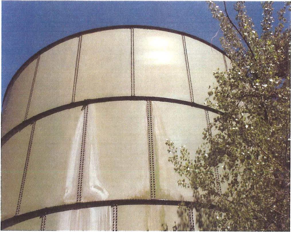
Seam Leak
