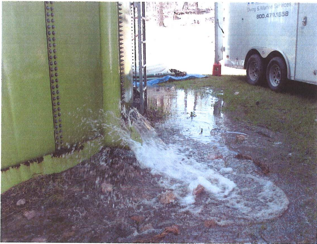
Tank at Overflow
