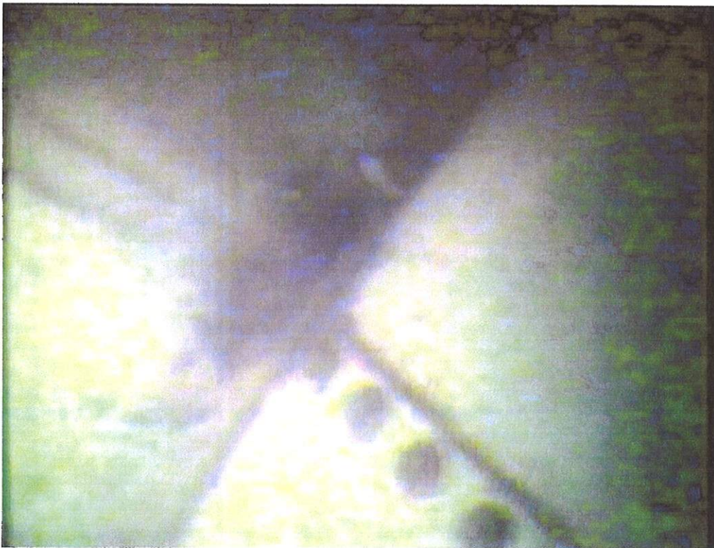
Floor to Wall Seam
