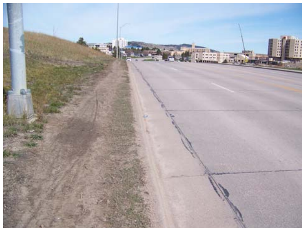
Shows lack of shoulder to serve as a buffer between foot- and vehicle traffic.
