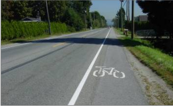
Figure 11. Shoulder bikeways are delineated with a fog line, and can use pavement stencils and signs.
