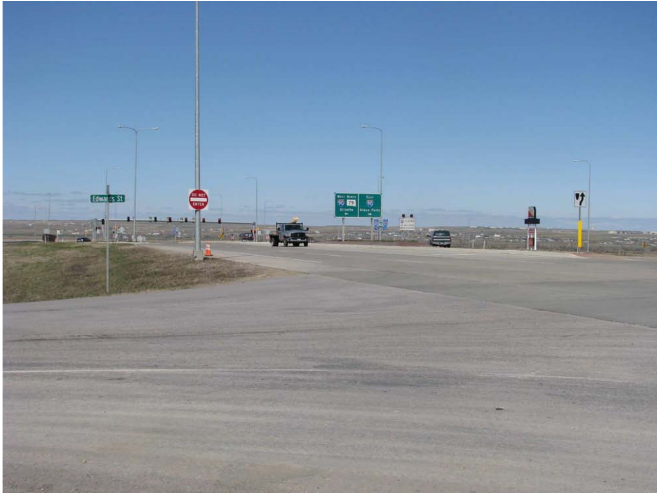
View looking towards north to Elk Vale DOT bridge over I-90 while standing at corner of Edwards & Elk Vale Rd.
