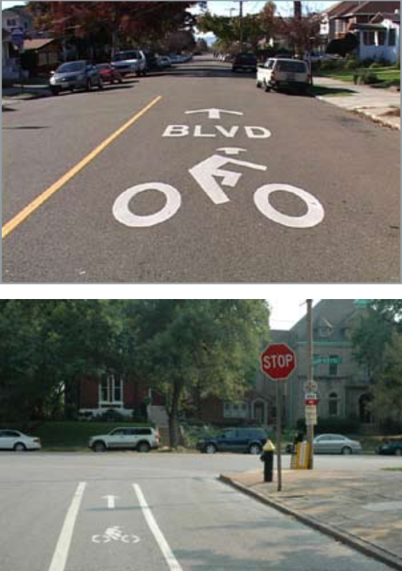
Bicycle boulevards in Berkeley (top) and Saint Louis (above). These streets parallel arterials and provide priority environments for bicycle transportation. Primary investments include removing hazards and providing pavement markings and signage. Bicycle boulevards may use sharrow (shared lane) pavement markings or bike lanes.
