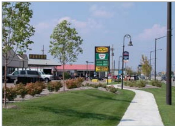
South Locust corridor in Grand Island, Nebraska used both a TIF district and a BID to develop and maintain right-of-way enhancements.
