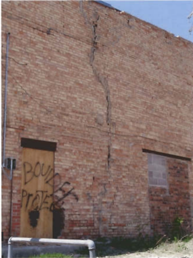
EAST WALL WITH CRACK
