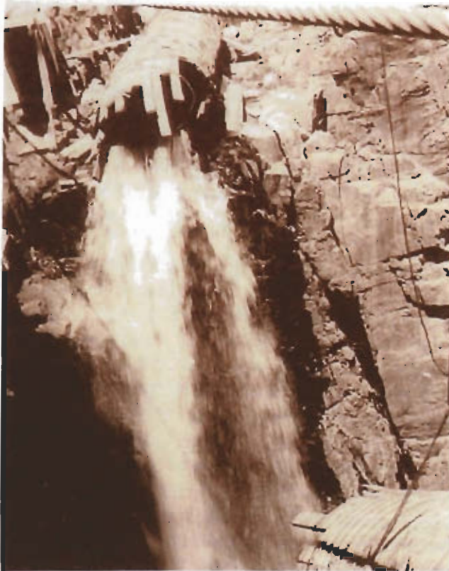
A common problem with the flume was leaks and damage because of weather or weak construction.
