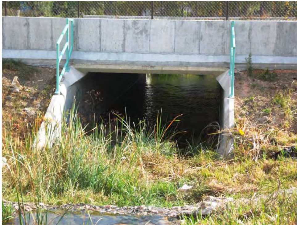
Element 17: Reservoir Road Box Culvert Inlet
