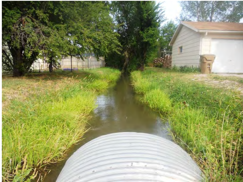
H6: Hawthorne Ditch looking downstream at Plateau Lane
