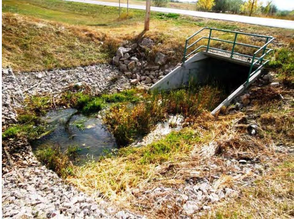
Element 17A: Longview Road Box Culvert Inlet
