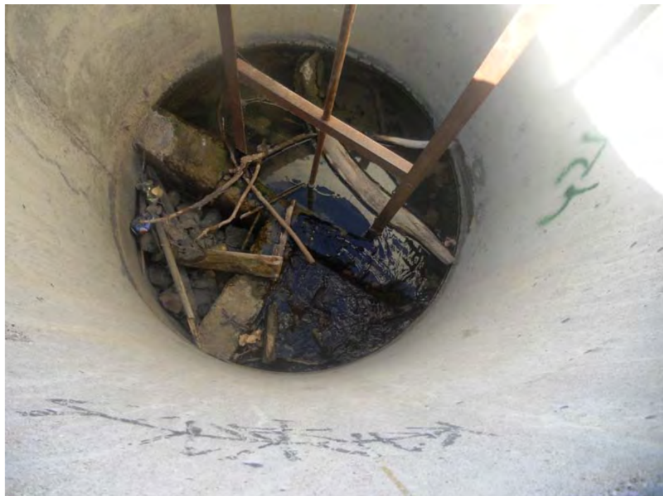
Detention Pond 102: Inside of Riser
