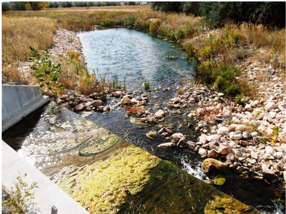
Element 20&21: Looking Downstream from Highway 44 Box Culvert
