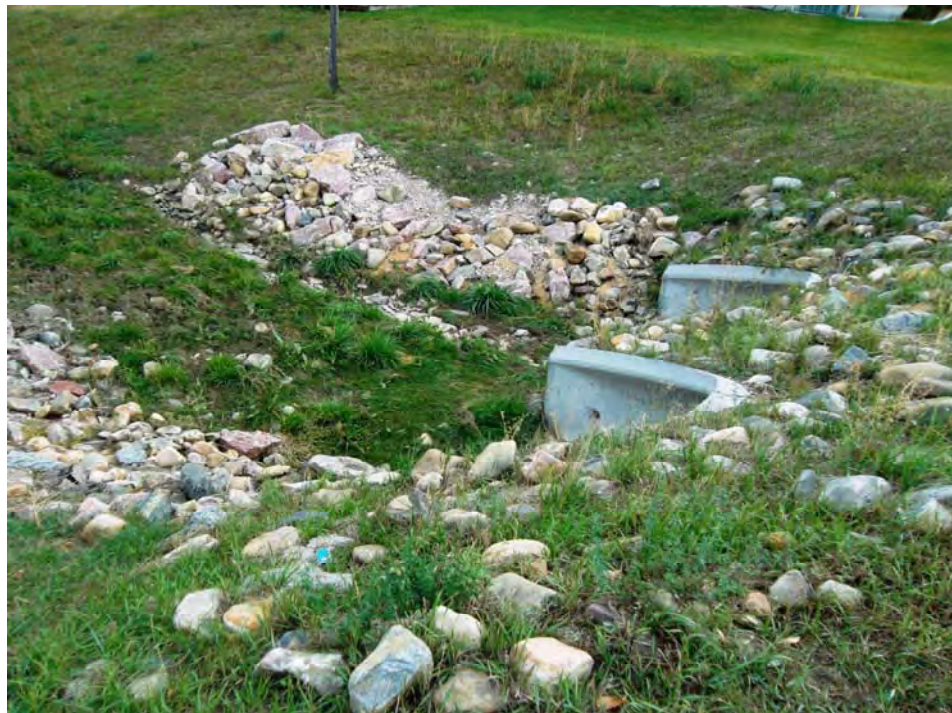
Element 10: Culvert Inlet End at Avenue A
