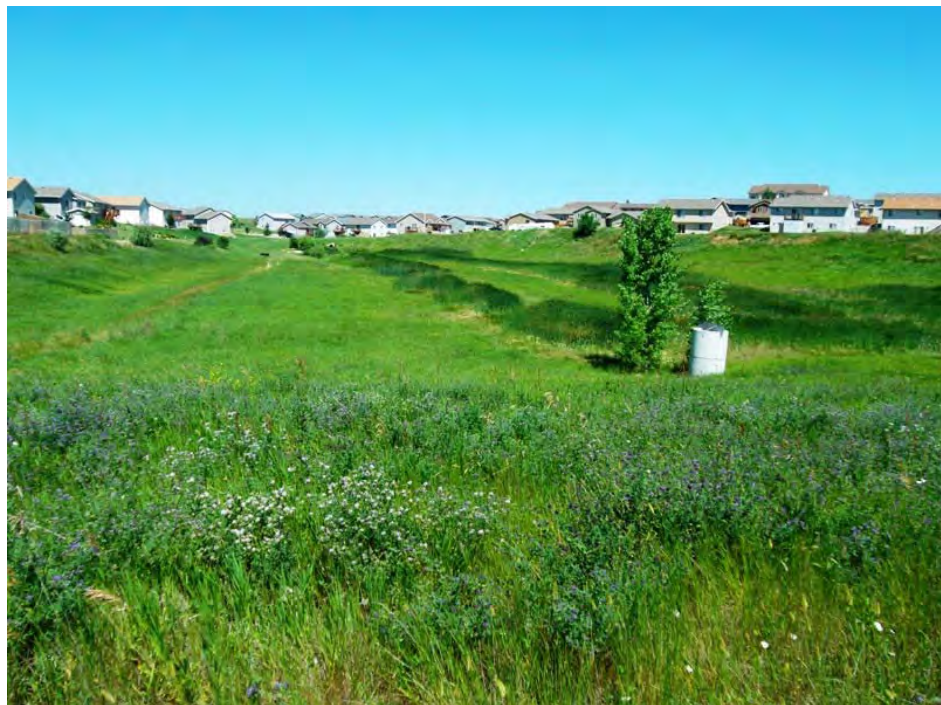
Element 8: Looking North from Top of Pond 100, Pond Riser is in Foreground
