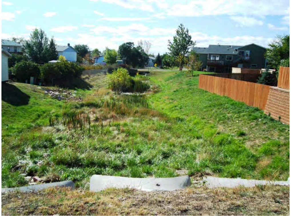
Element 6: Inlet End of Culverts Under Avenue A
