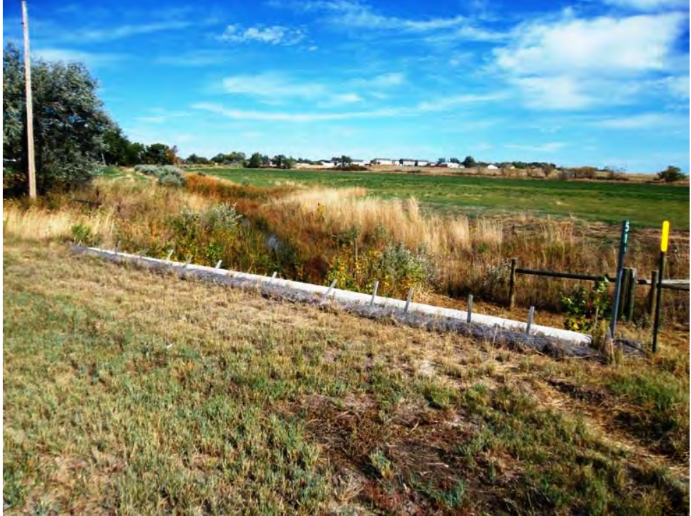
Element 19&20: Looking Upstream from Highway 44 Box Culvert
