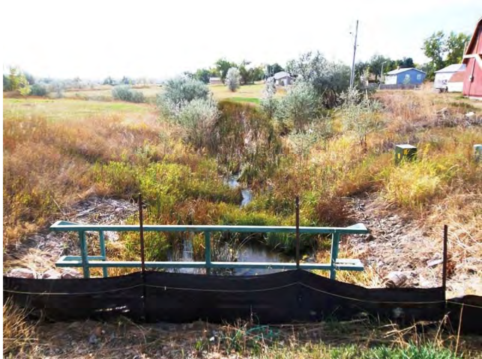
Element 18: Looking Downstream from Longview Road
