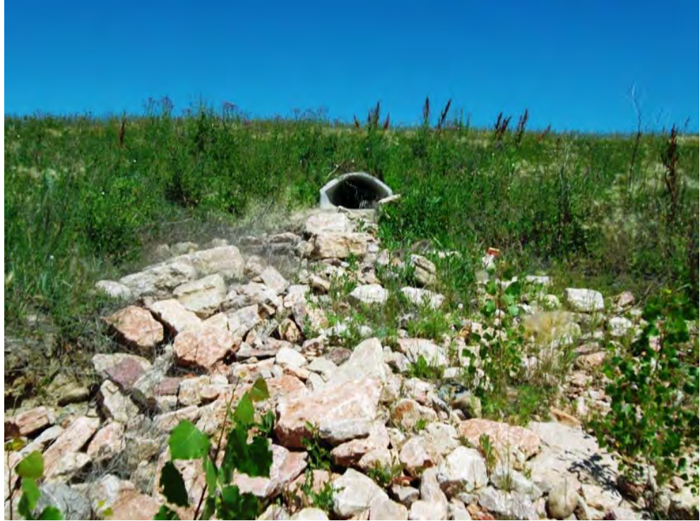
Element 3: Outlet End, Looking Downstream from Homestead Street
