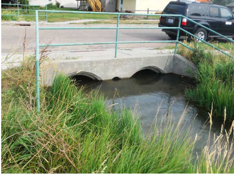
H7: Hawthorne Ditch at Sprucewood Street (inlet end is shown)
