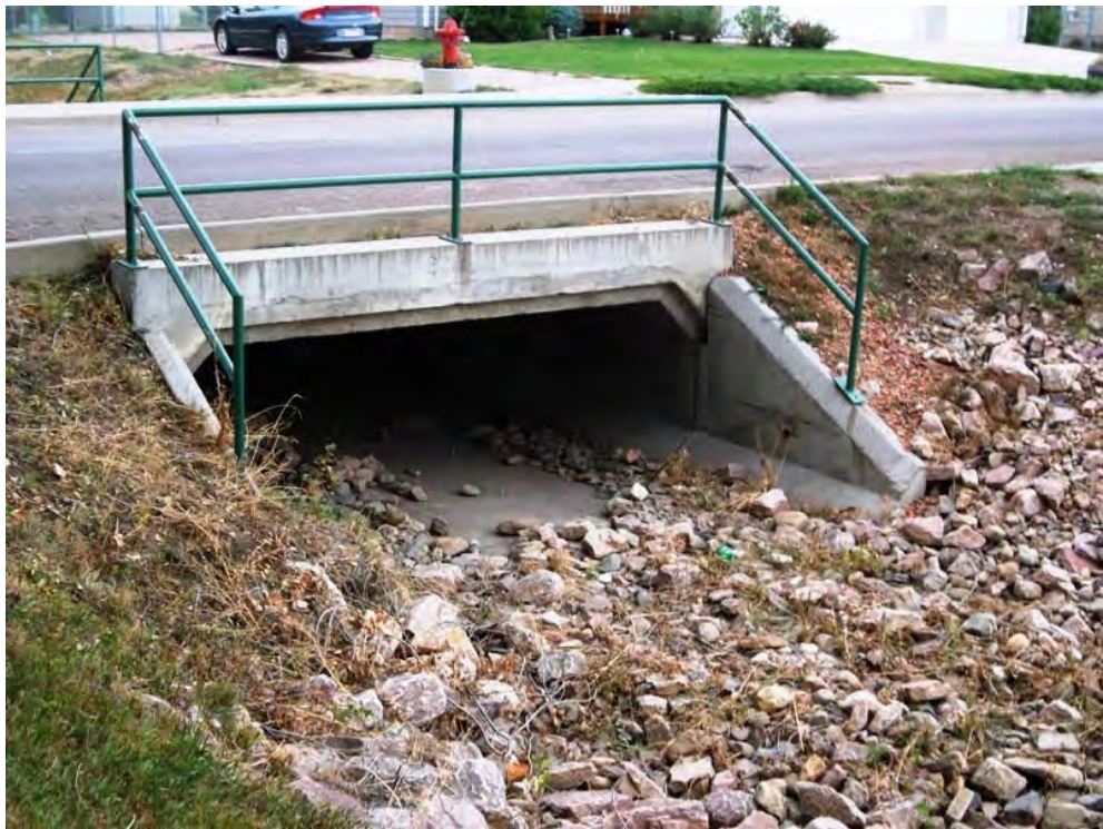
Element 14: Leroy Street Looking Upstream
