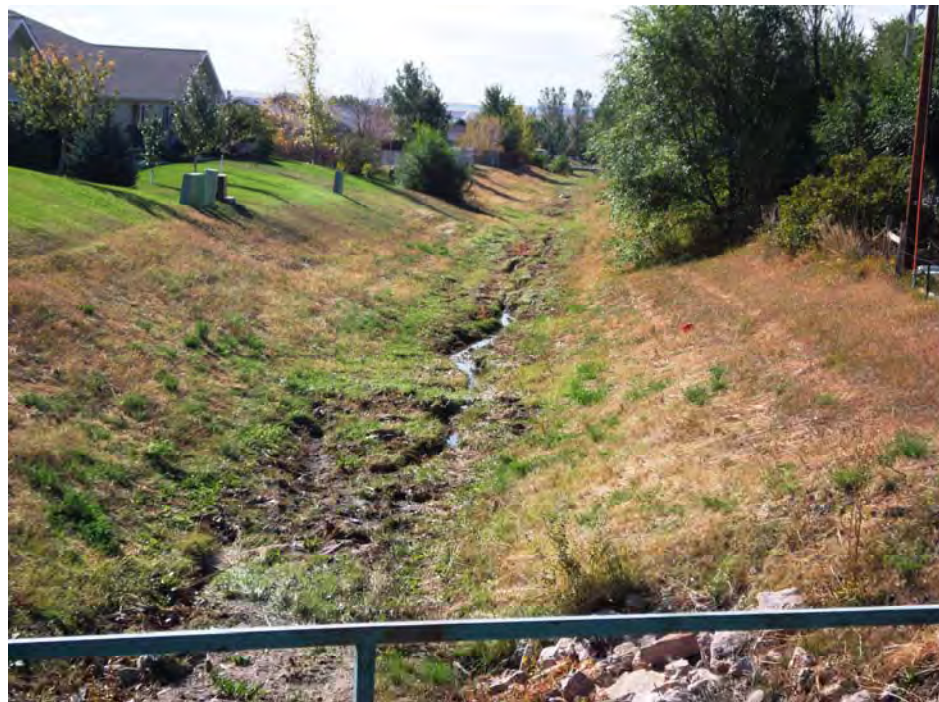
Element 14: Looking South from Twilight Drive Box Culvert
