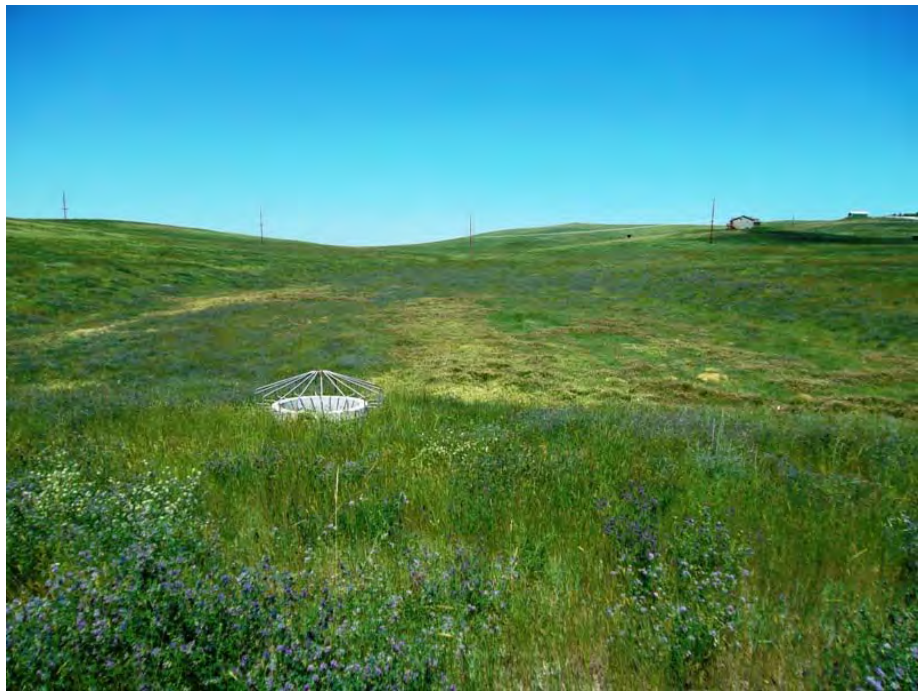
Detention Pond 103: Looking North from Top of Dam, Riser in Foreground
