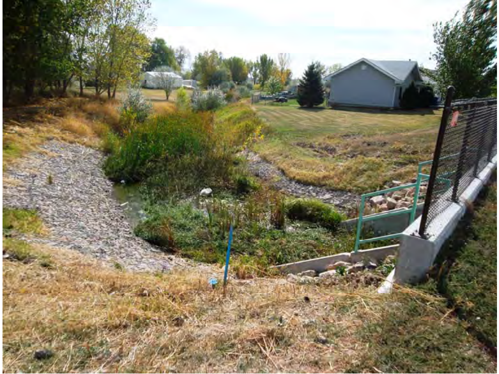
Element 17A: Looking Downstream from Reservoir Road
