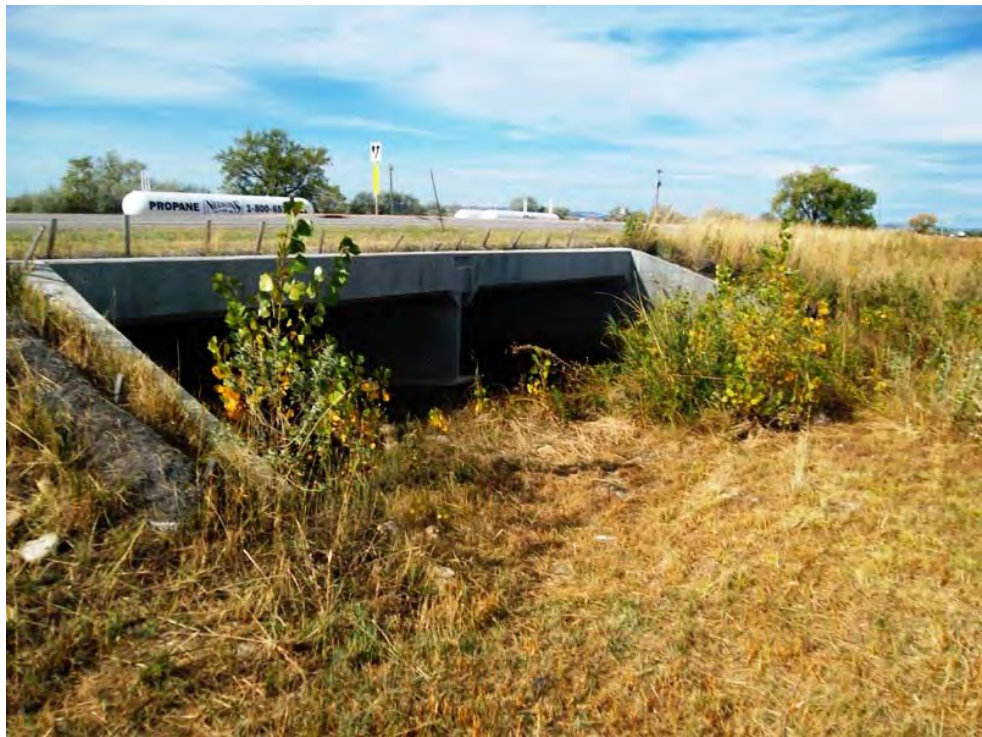
Element 20: Highway 44 Box Culvert Inlet
