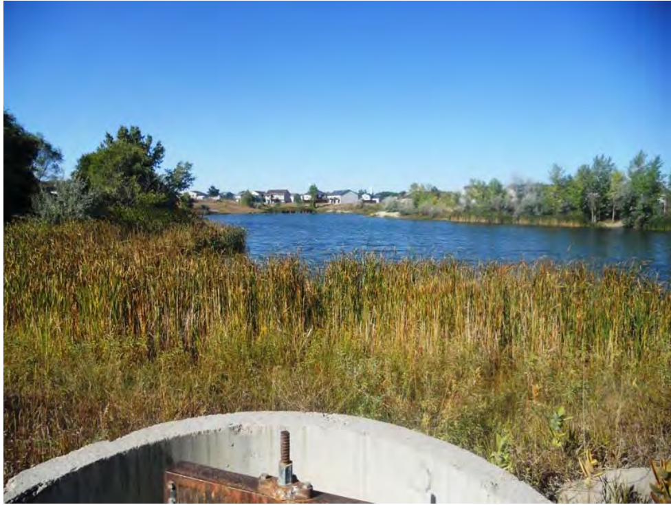
Detention Pond 102: Looking North from Dam, Riser in Foreground
