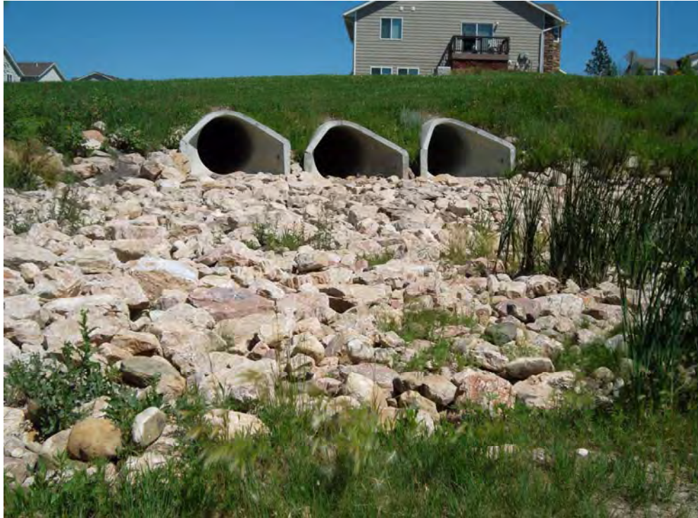
Element 8: Outlet End of Pipes Under Pedestrian Path
