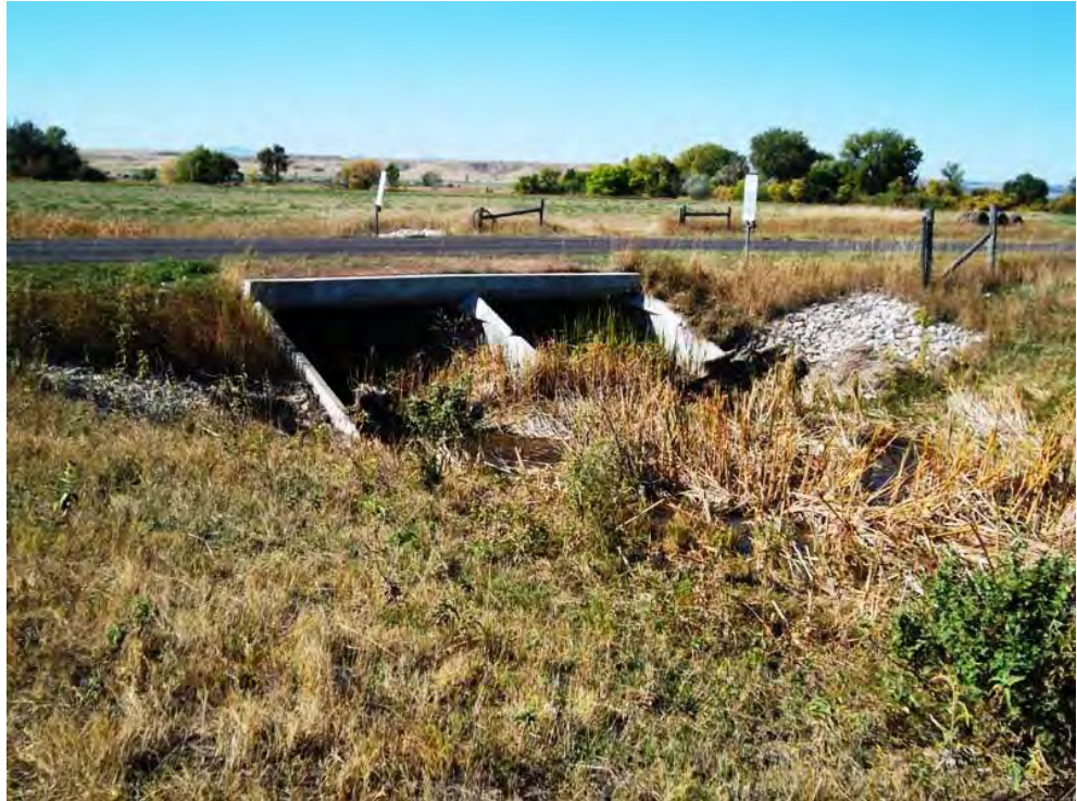
Element 22: Green Valley Drive Box Culvert Inlet
