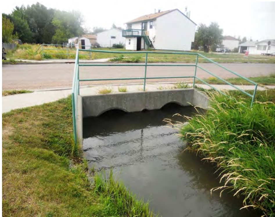
H8: Hawthorne Ditch at Sprucewood (outlet end is shown)
