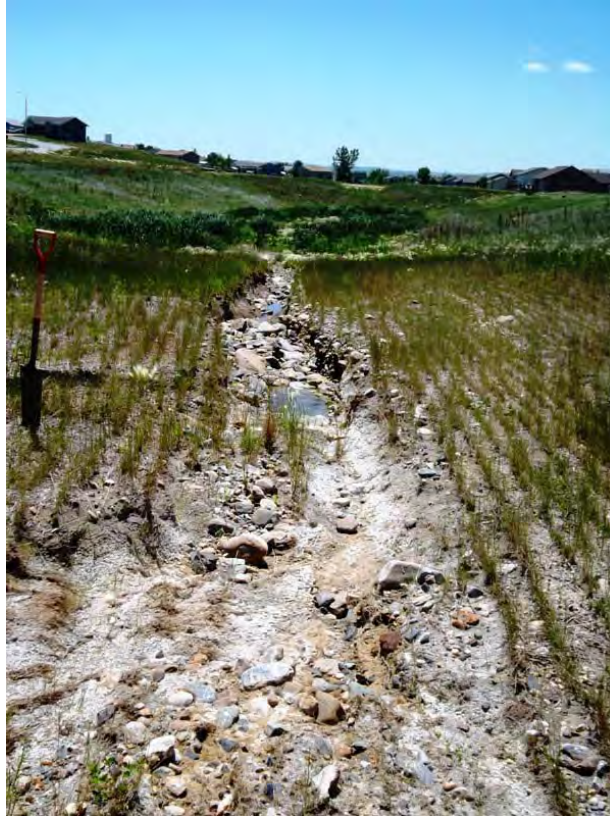
Element 2: Looking South into Bottom of Pond 104
