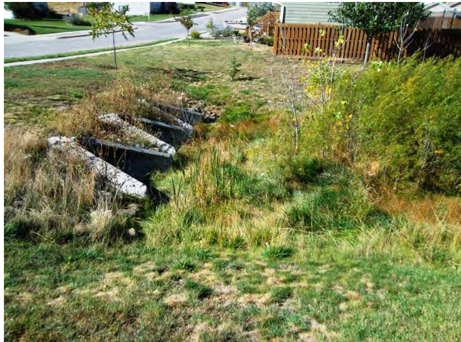
Element 6: Inlet End of Culverts Under South Pitch Drive
