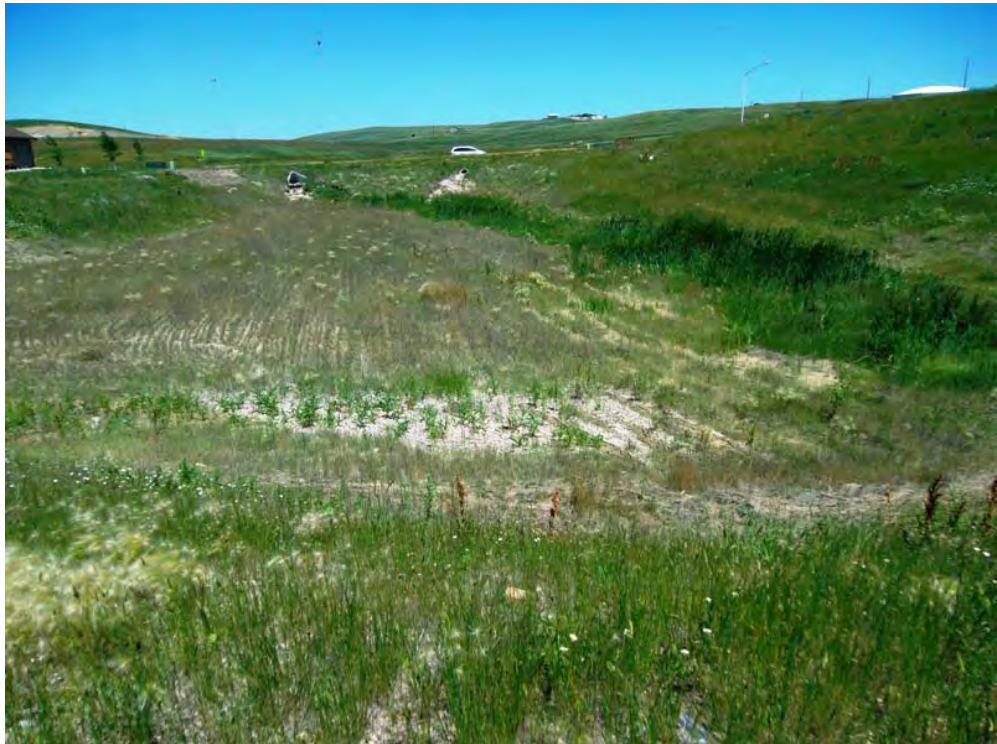
Detention Pond 101: Looking North from Dam
