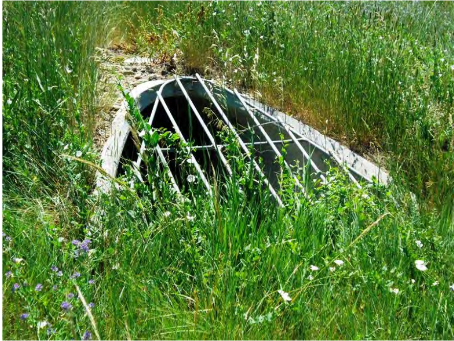
Detention Pond 103: Secondary Pipe Inlet
