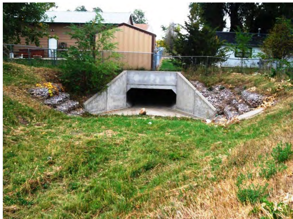
Element 15: Albert Lane Box Culvert Inlet
