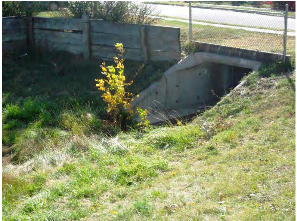
Element 7: Plateau Lane Box Culvert Inlet
