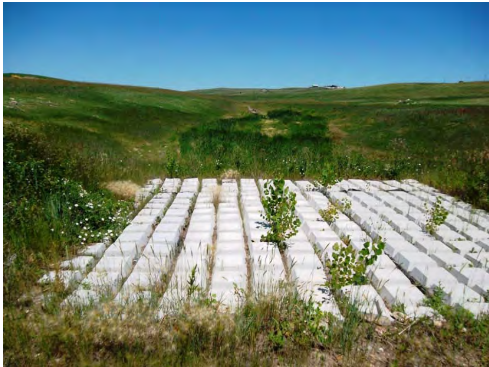
Detention Pond 103: At Spillway looking North
