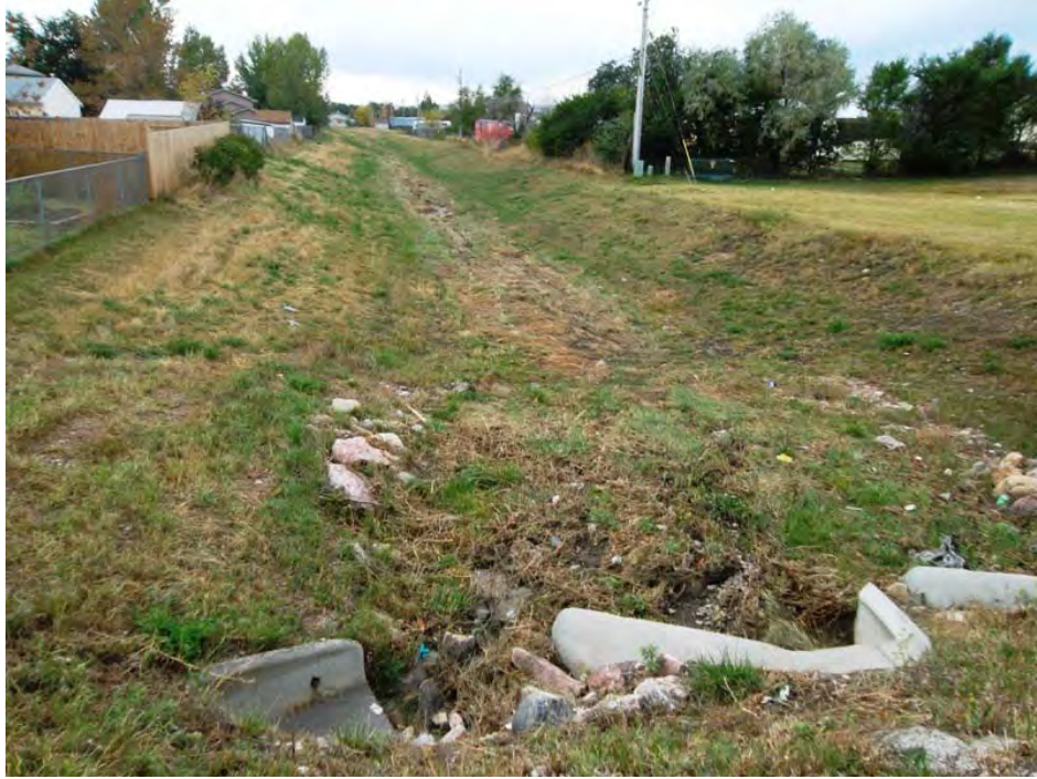
Element 10: Looking Downstream from Avenue A
