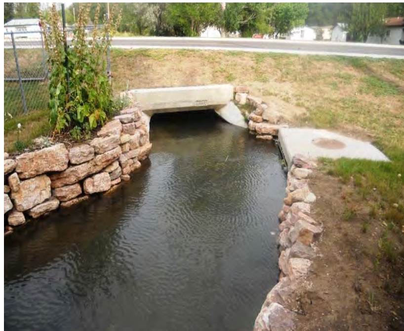
H10: Hawthorne Ditch at Reservoir Road (inlet end is shown)
