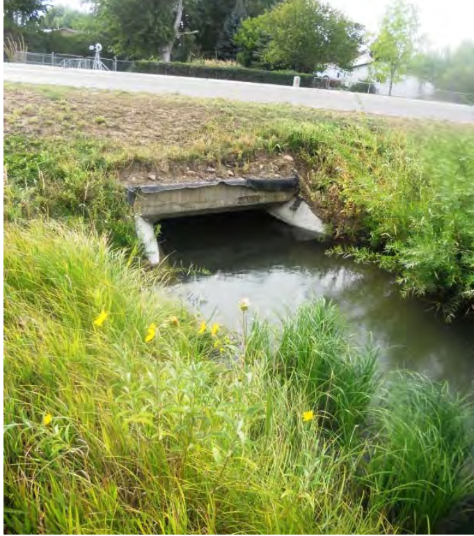
H11: Hawthorne Ditch at Reservoir Road (outlet end is shown)
