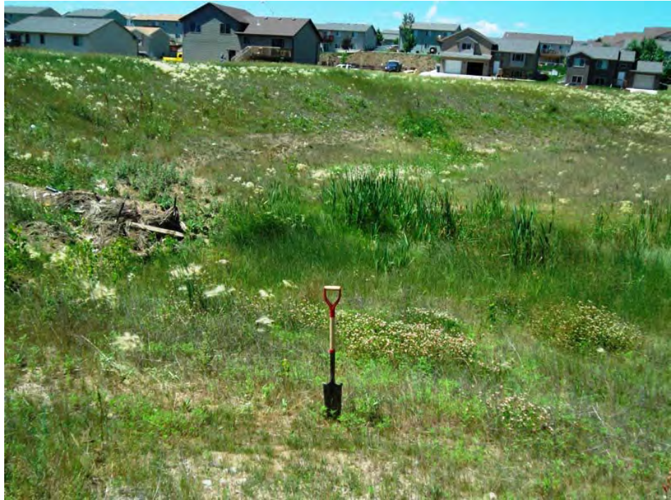
Detention Pond 101: Looking West, Note Outlet Pipe covered with Debris
