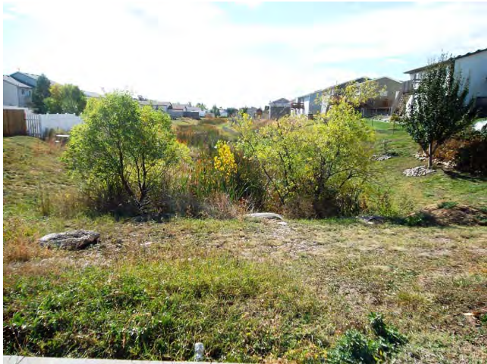
Element 6: Looking Downstream of South Pitch Drive
