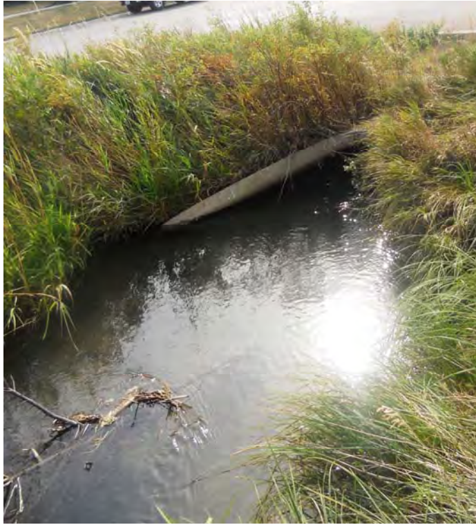
H3: Hawthorne Ditch at Reed Court (outlet end is shown)
