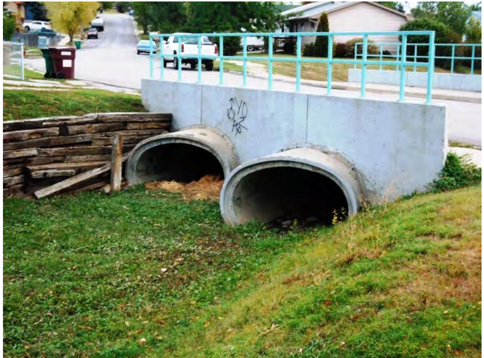
Element 11: Plateau Lane Culvert Inlet End
