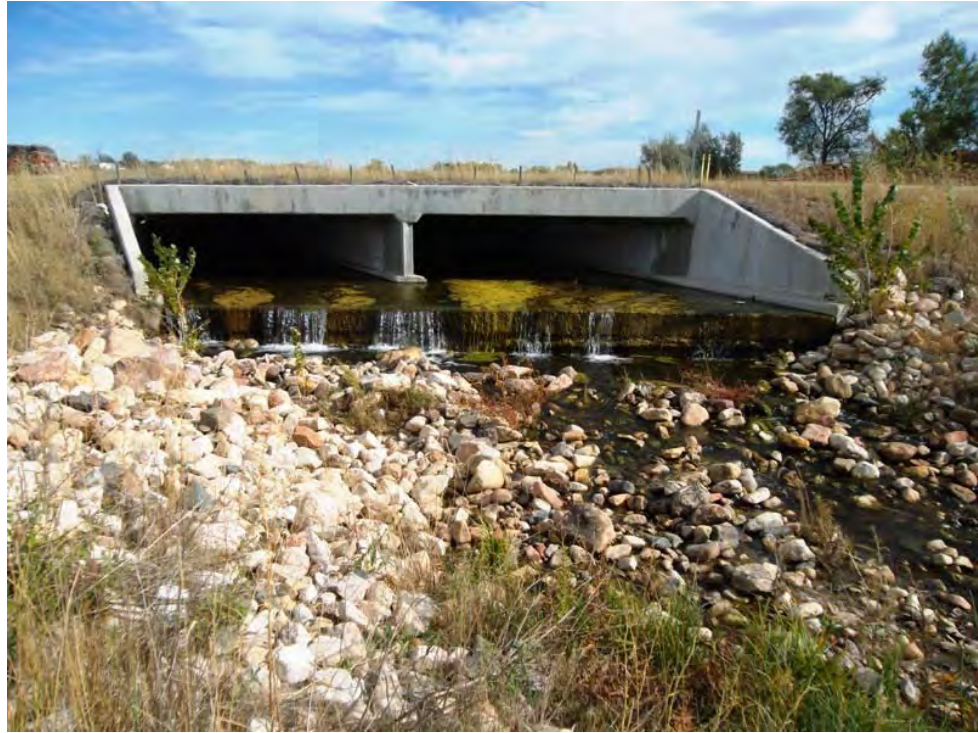
Element 20: Outlet of Highway 44 Box Culvert
