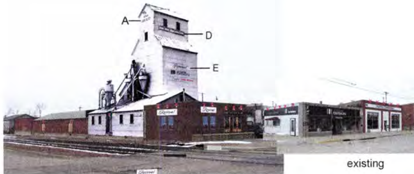
view from 5th street
