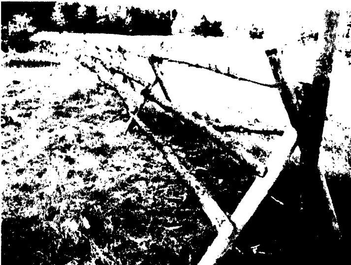
Figure 1 – Representative style for north fence.
