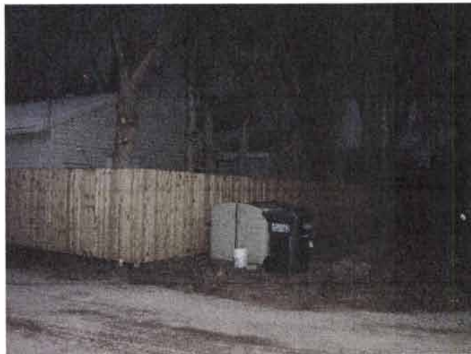
South west corner of property looking north easterly
