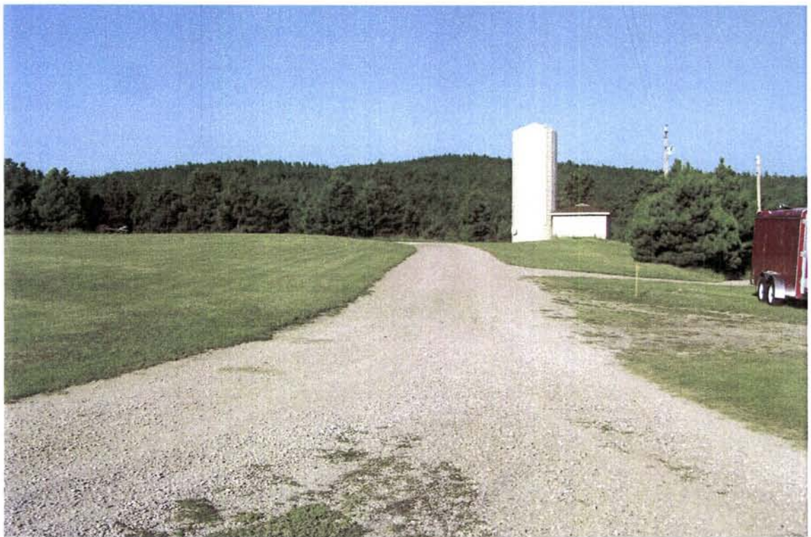
Access Easement – looking west, from east end of lot, towards Strato Rim Drive
