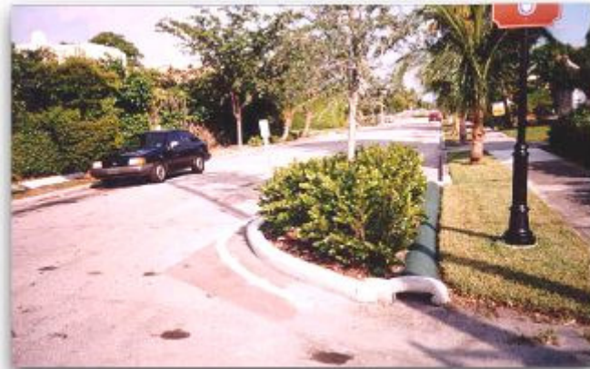
Illustration of a Chicane
