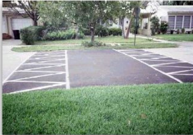
Illustration of a Speed Table
