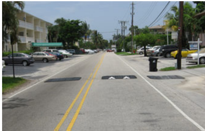
Illustration of a Speed Cushion
