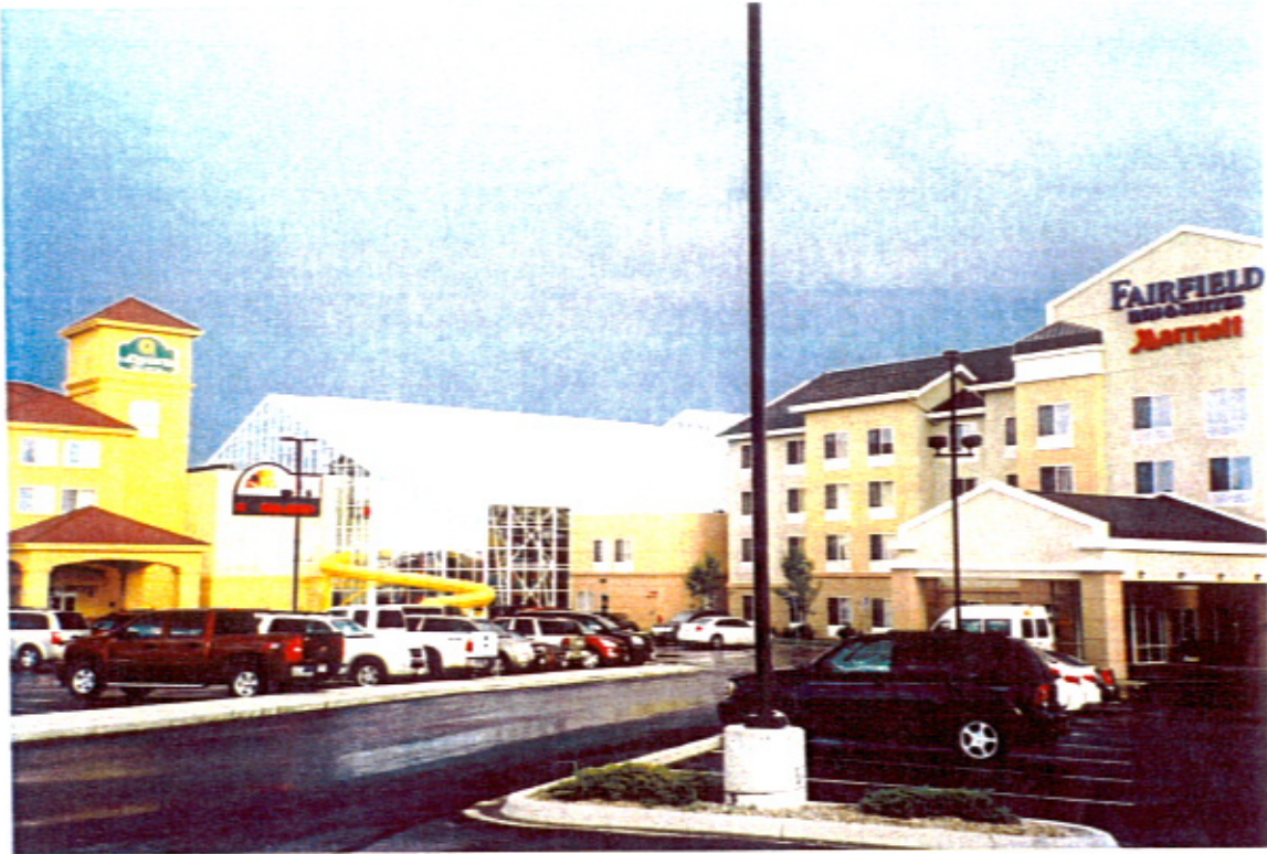
WaTiki Indoor Water Park & Fairfield Inn & Suites (view from the north – looking south)
