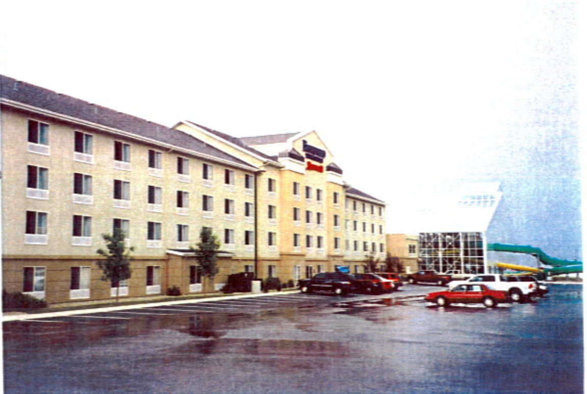
Fairfield Inn & Suites (south face of the building – view from the southwest – looking northeast)
