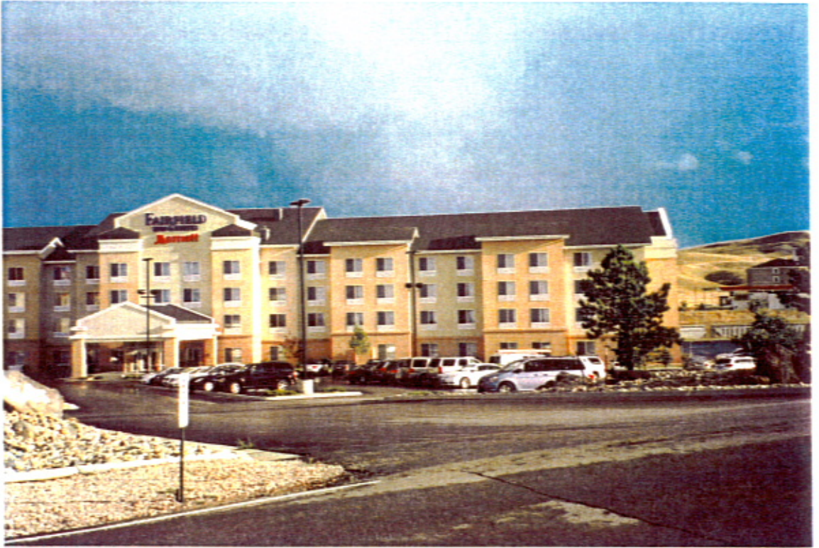
Fairfield Inn & Suites (west end of the facility – view from the north – looking south)
