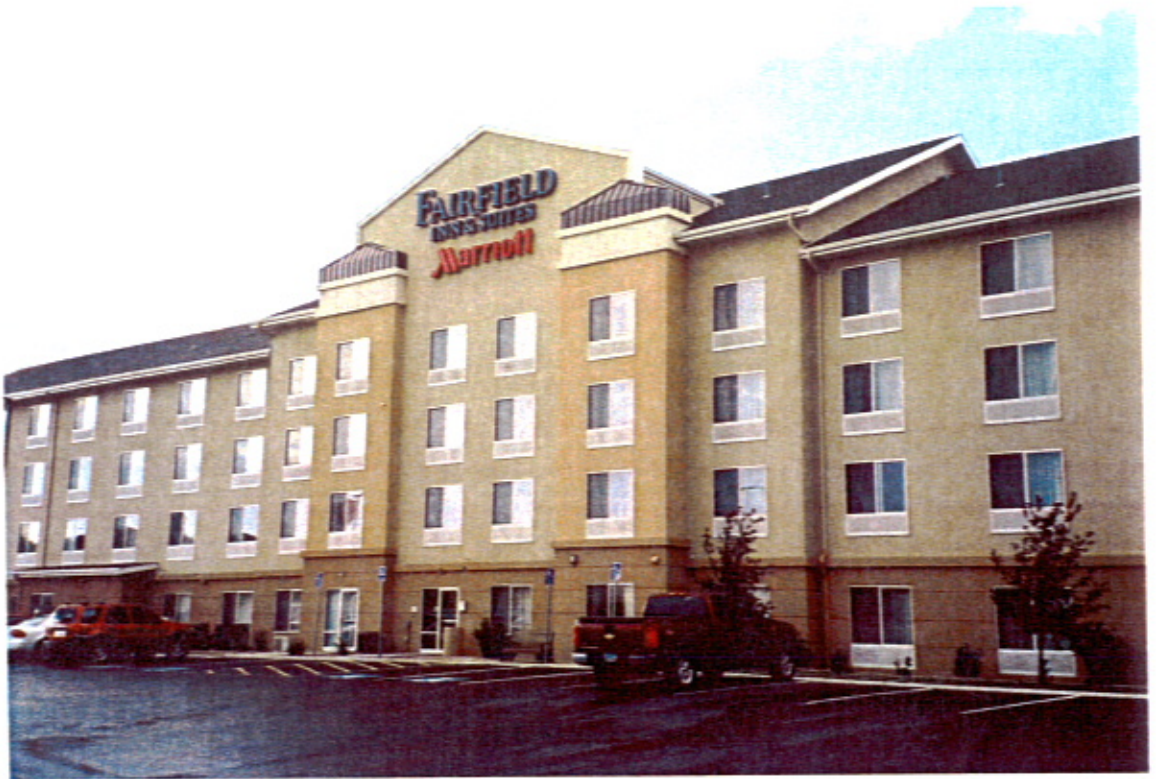
Fairfield Inn & Suites (rear of the building – view from the south looking north)
