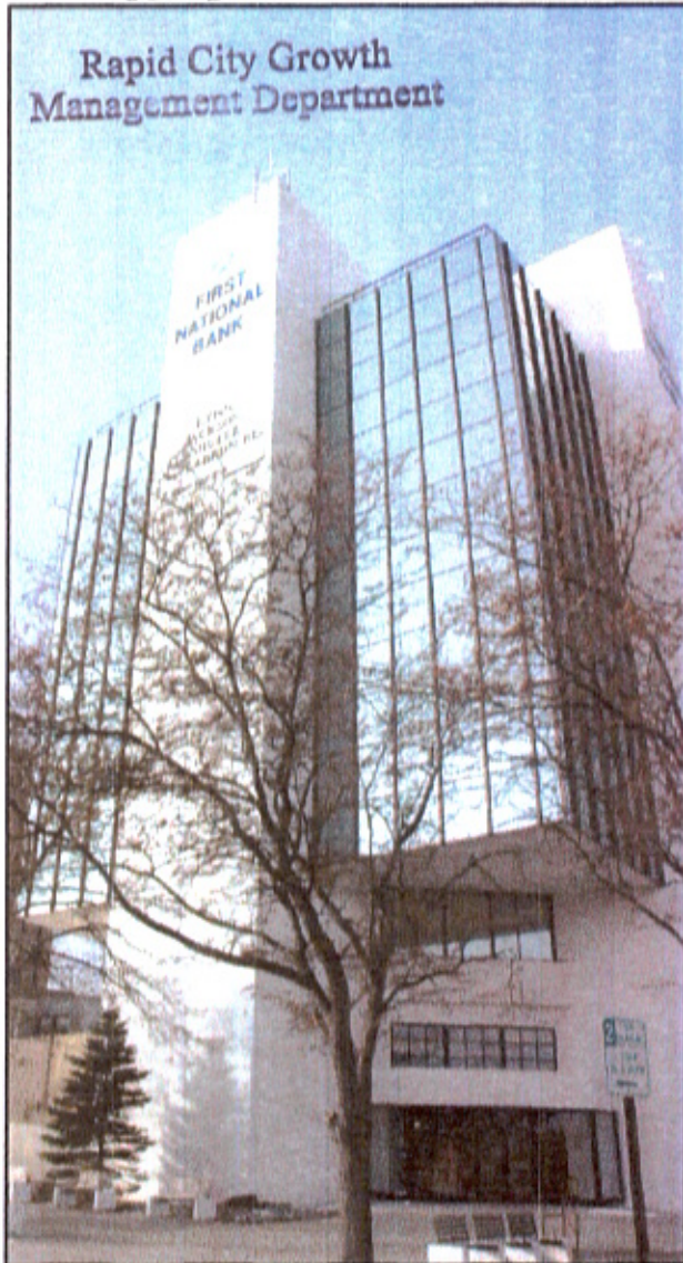
4 OVERALL TOWER PHOTO SCALE: NONE
