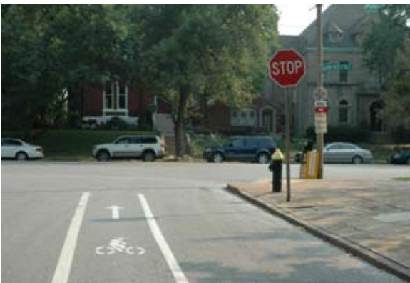
Bicycle boulevards in Berkeley (top) and Saint Louis (above). These streets parallel arterials and provide priority environments for bicycle transportation. Primary investments include removing hazards and providing pavement markings and signage. Bicycle boulevards may use sharrow (shared lane) pavement markings or bike lanes.
