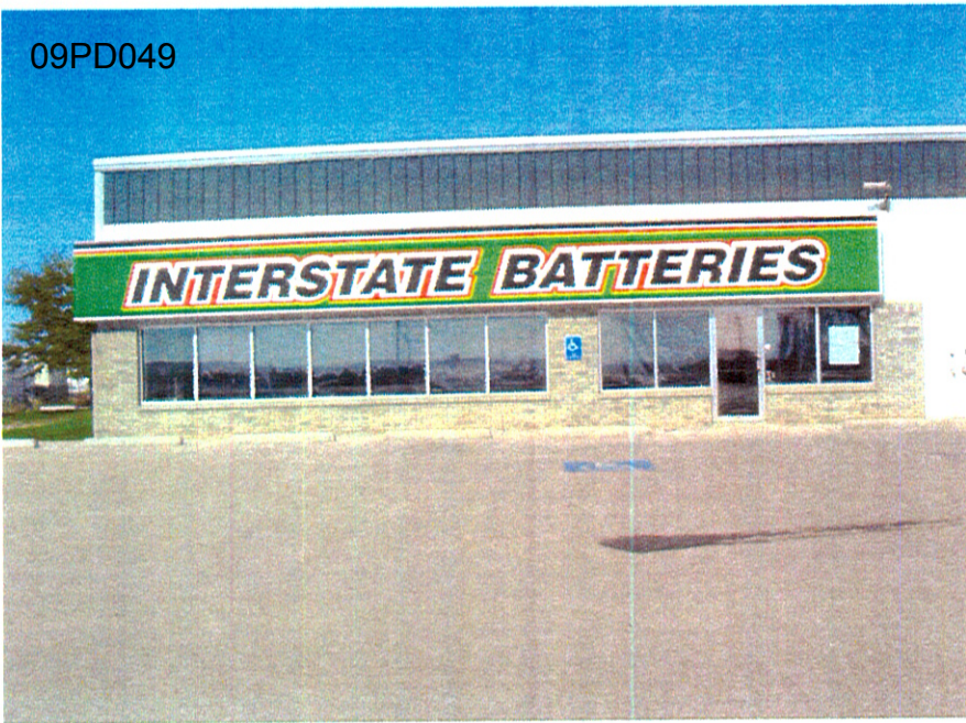
Existing Store Front
