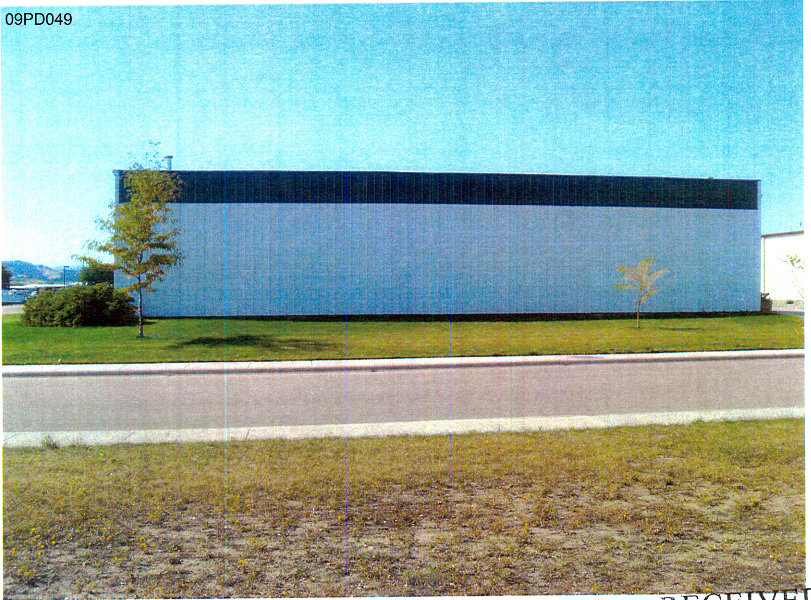
East Side of Building
