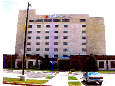
Photo 4 View of rear facade of hotel.
