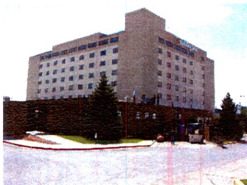
Photo 5 View of rear of hotel.
