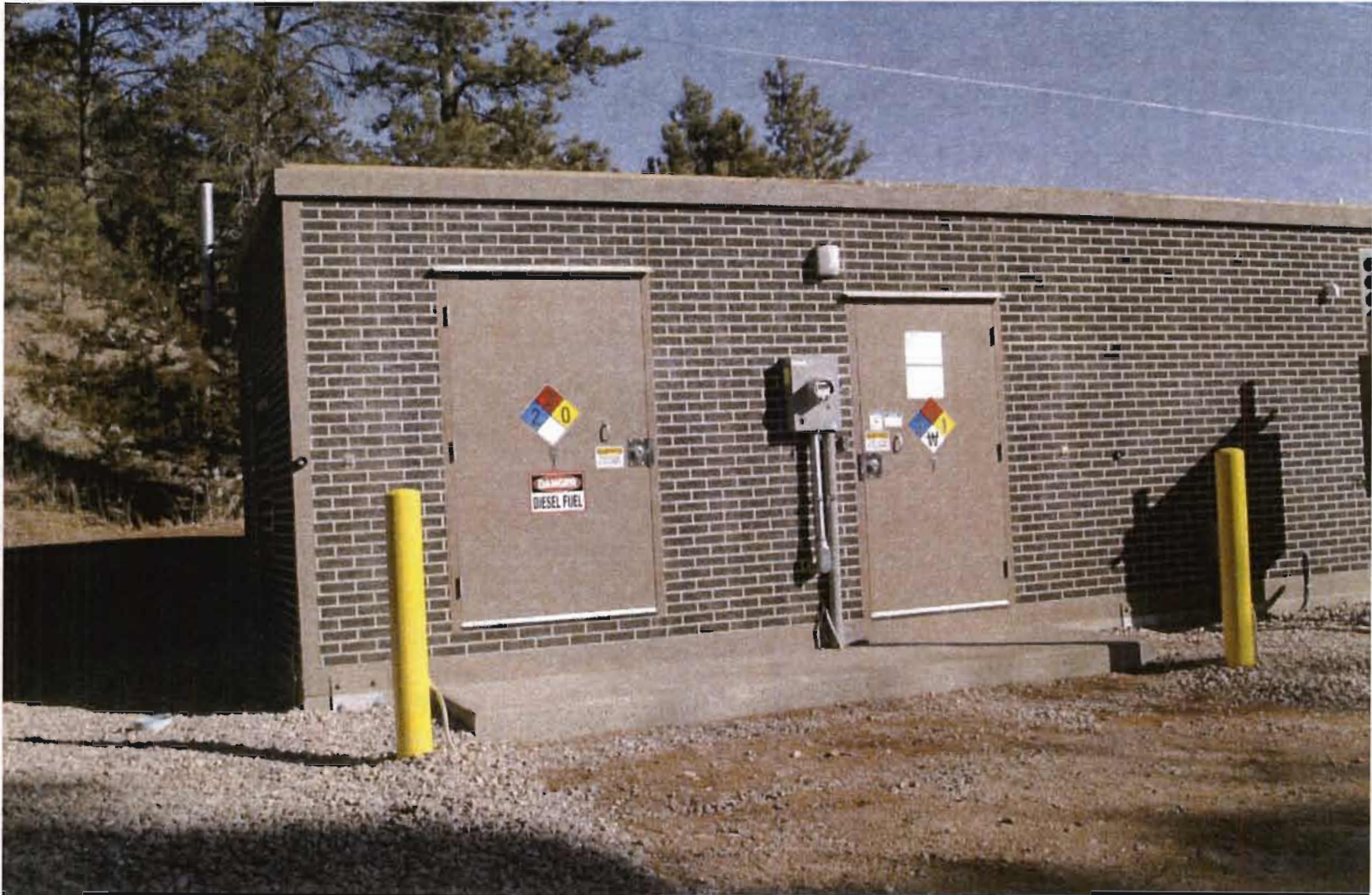
View of the brick communications shelter located just south of the monopole.
