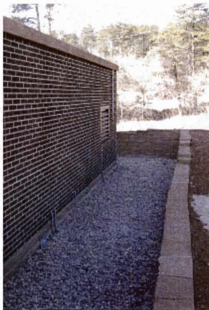
The berm on the west side of the communications shelter.
