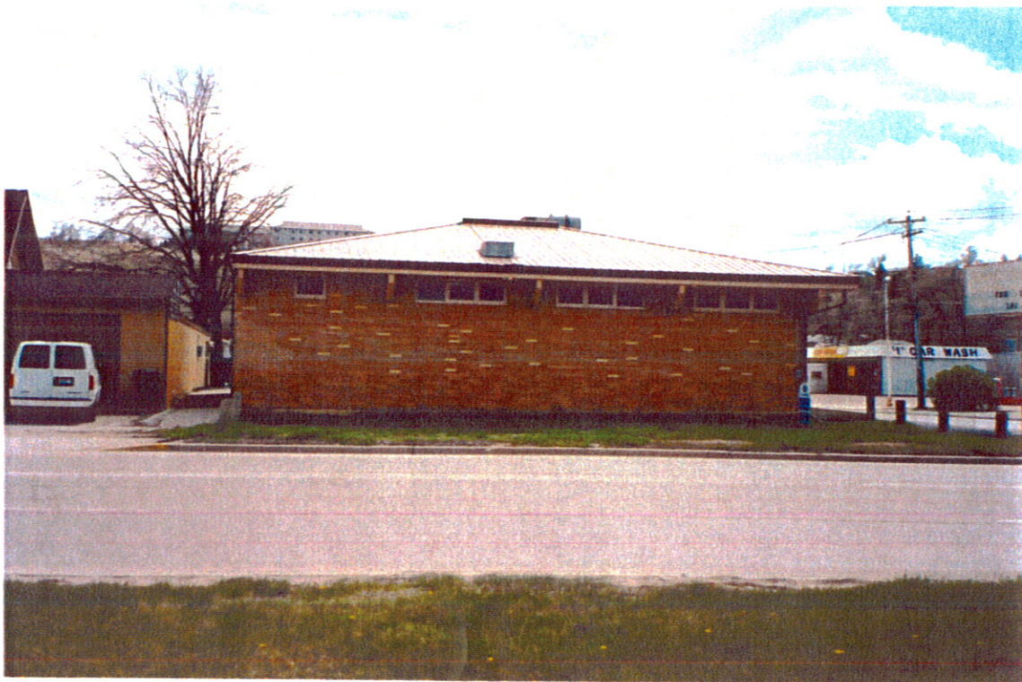
(north face of building – looking south)
