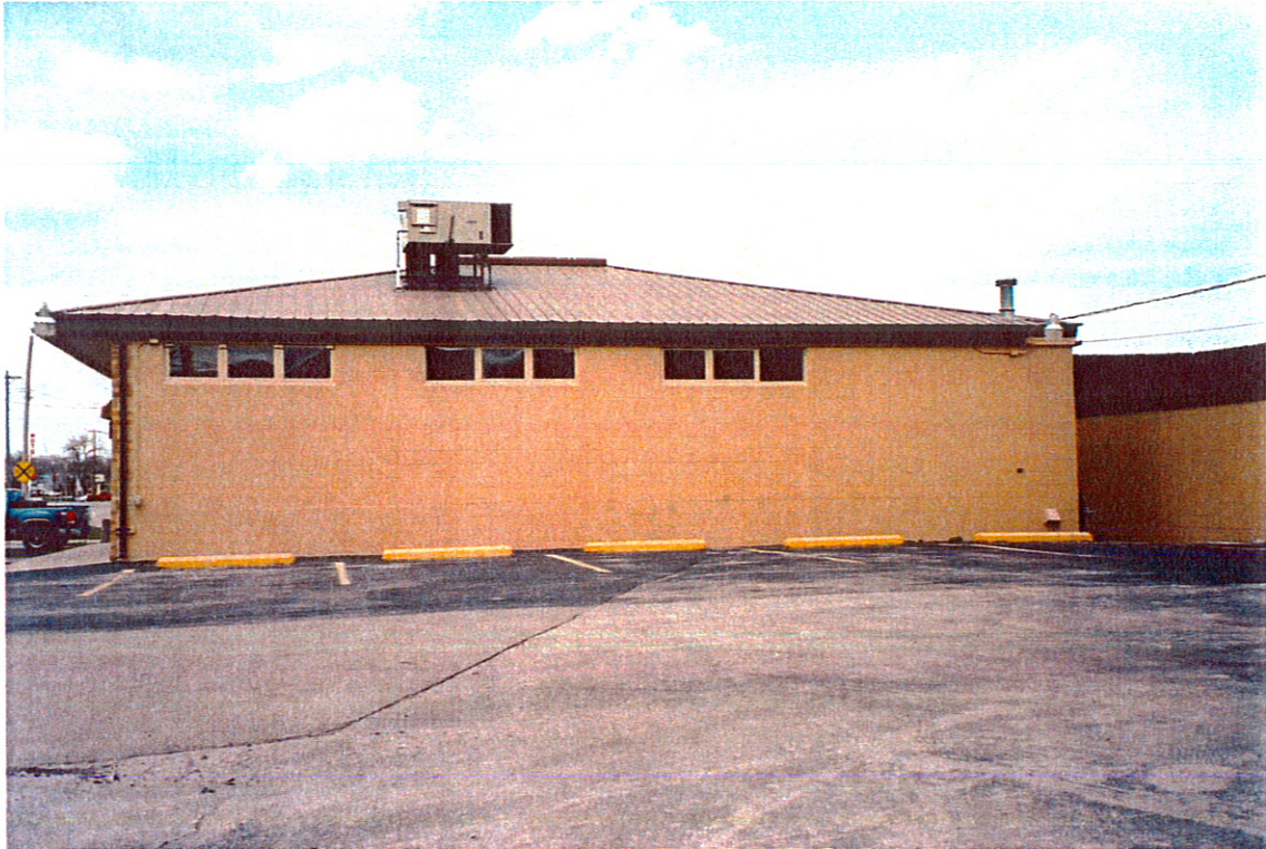
(south face of the building – looking north)
