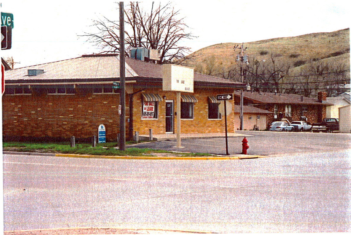
(north face of building – looking southeasterly)
