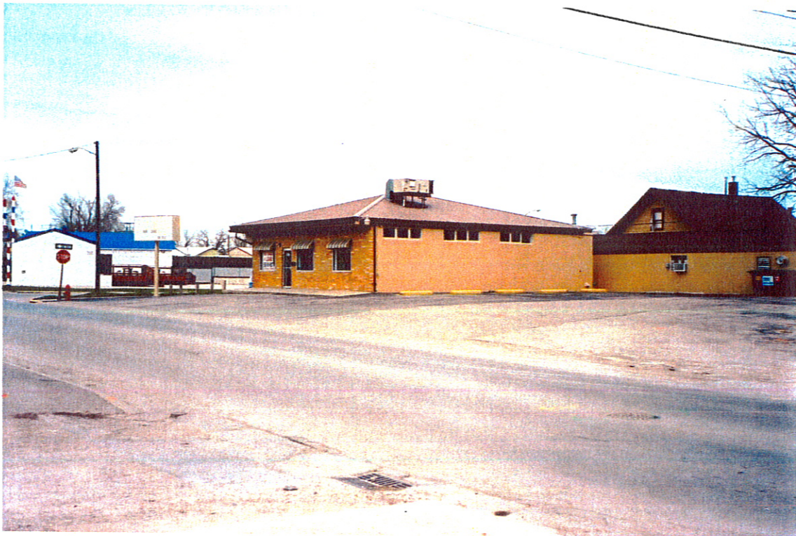
(southerly face of building – looking northeasterly)
