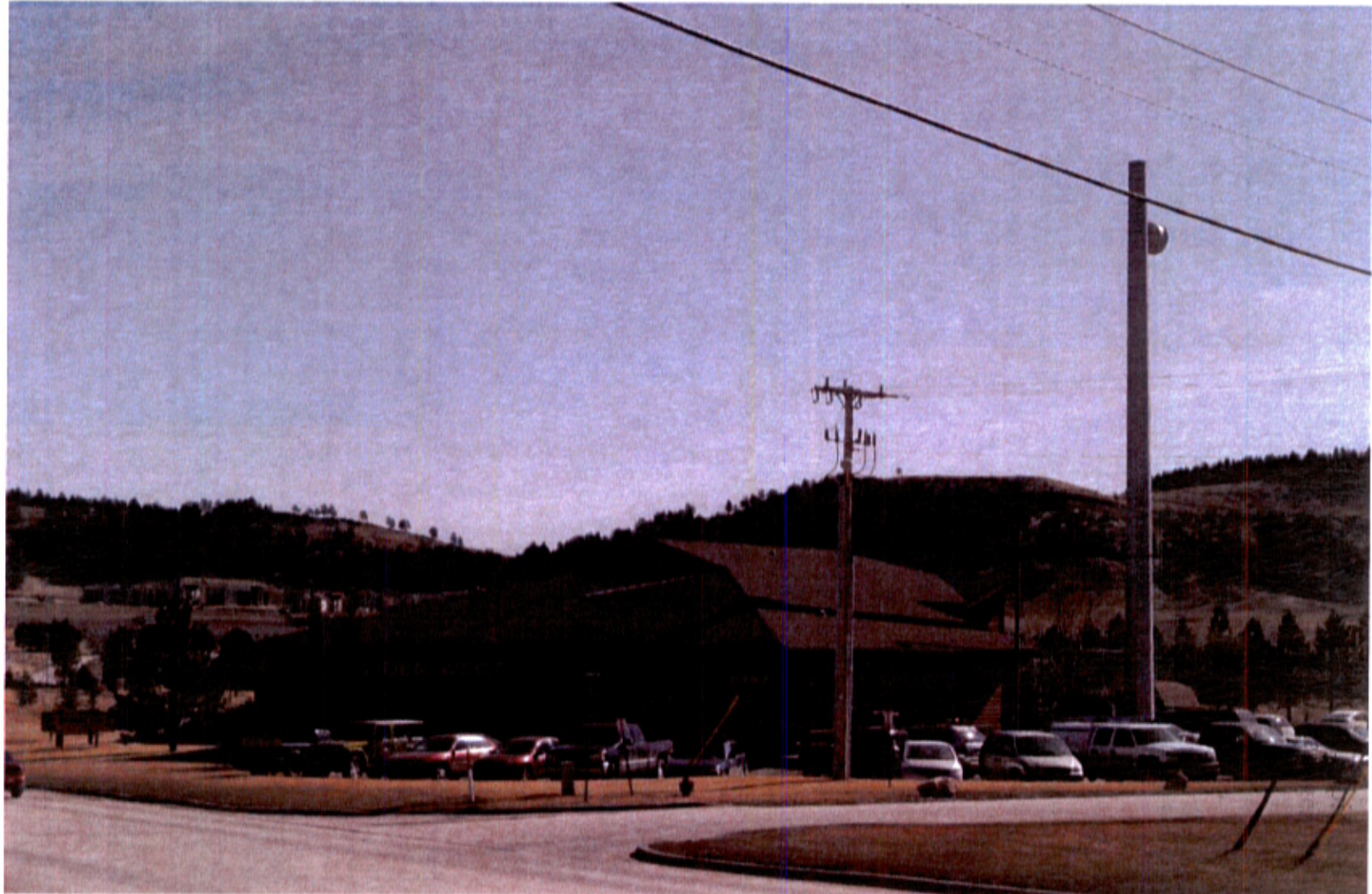
View looking southeast at the Golden West monopole and building.
