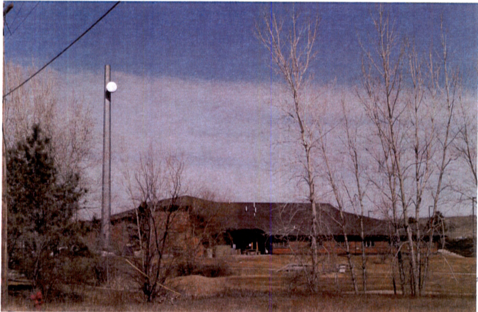
View looking north-northeast at the Golden West monopole and building.
