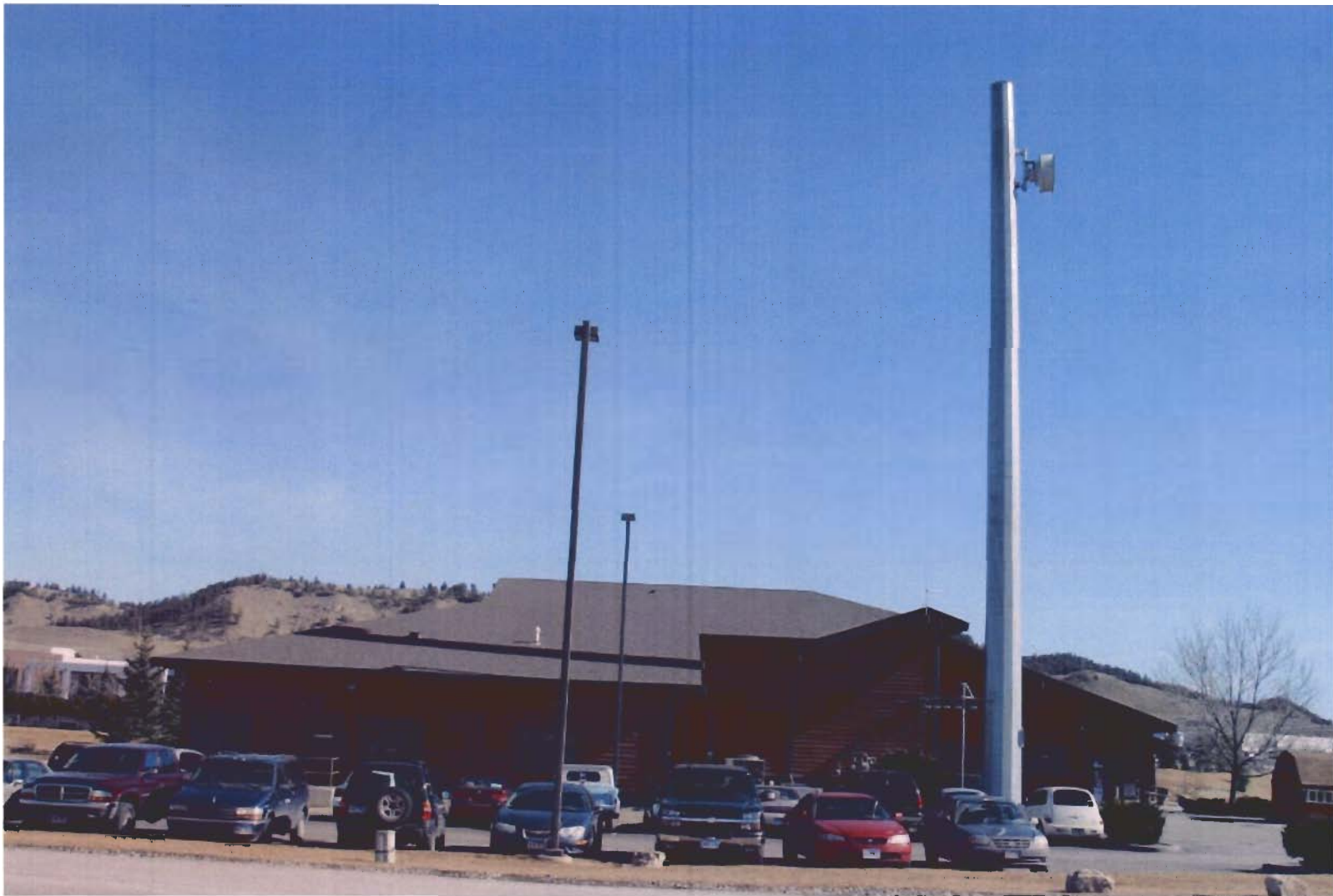
View looking east to 120' monopole.
