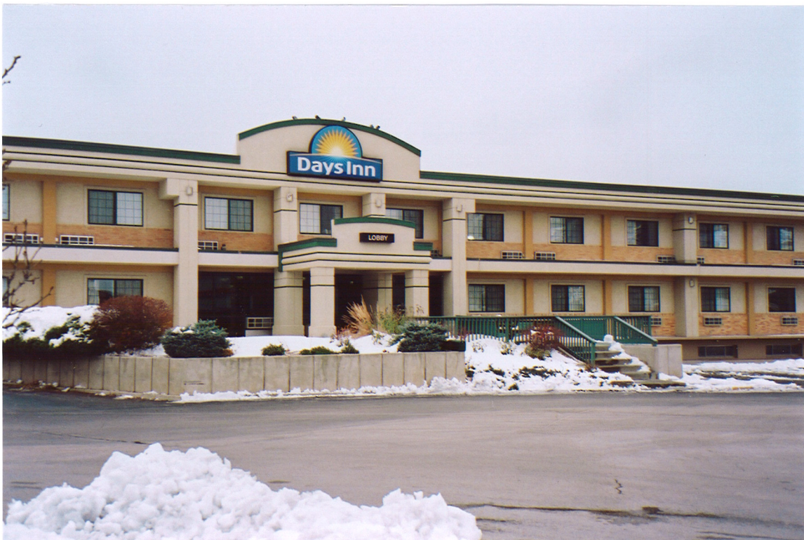
Concrete Retaining Walls & Wood Fencing on North Side of Building
