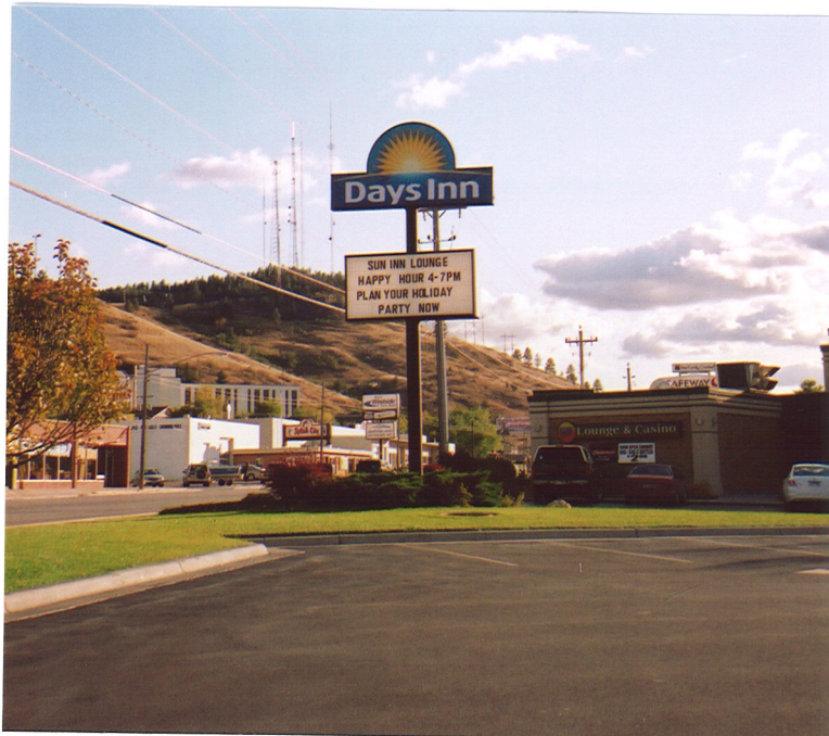
Days Inn Pole Sign northeast of building and Lounge & Casino sign on north face of building (sign details on following page)
