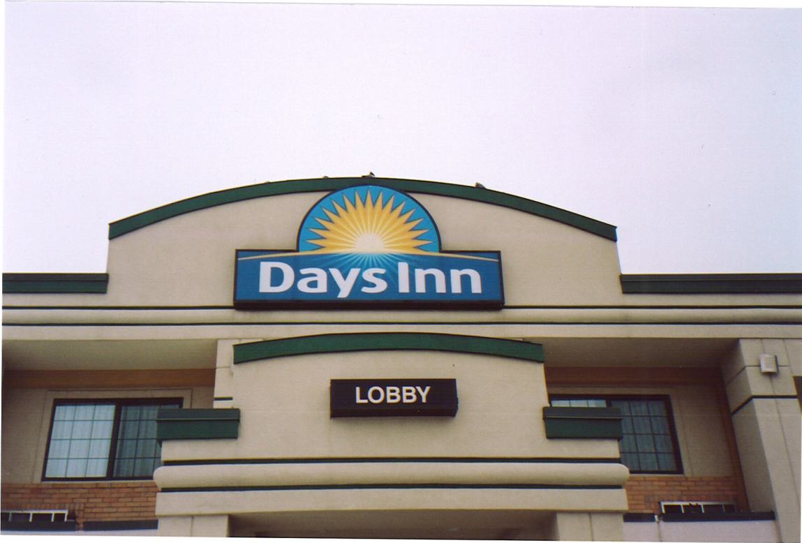
Days Inn Sign – north face of building over entrance (approximately 6' tall x 12' wide)
