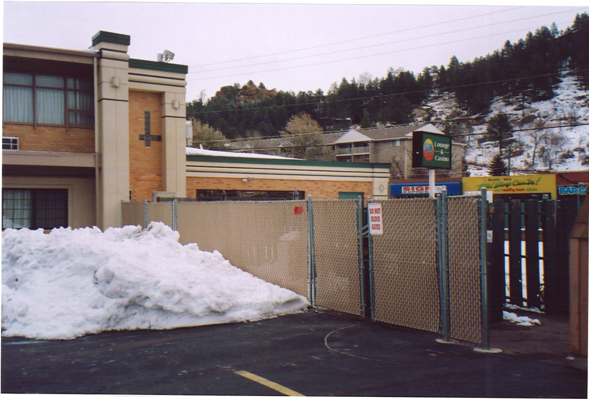
Refuse Enclosure (East End of South Parking Lot – Enclosed by Chain Link with Screening on West & Wood Fence on South)
