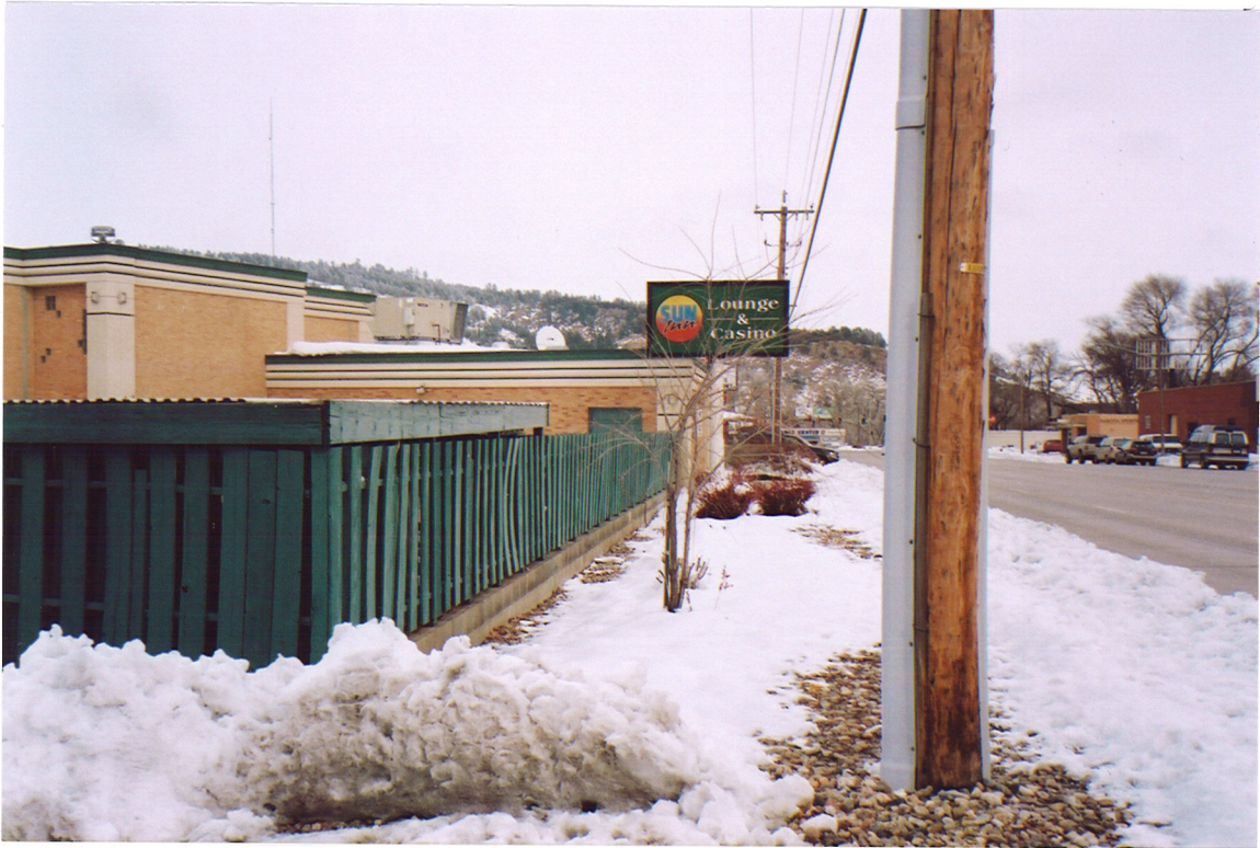
4' tall Wood Fence on 2' tall Retaining Wall (east side of the property)
