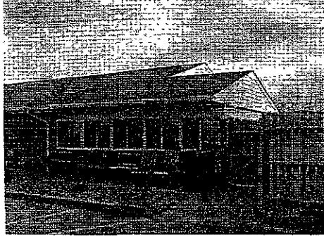
EXISTING NORTH FACE OF WEST WING TO RECEIVE BUILDING ADDITION - TEMPORARY EGRESS @ EXISTING WINDOW - EXISTING FENCE TO BE REMOVED
