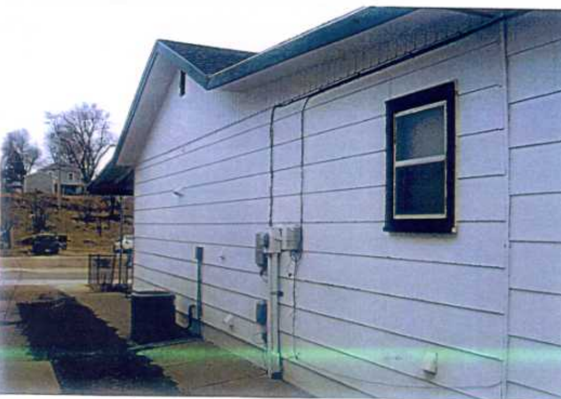
NORTH SIDE OF HOUSE
