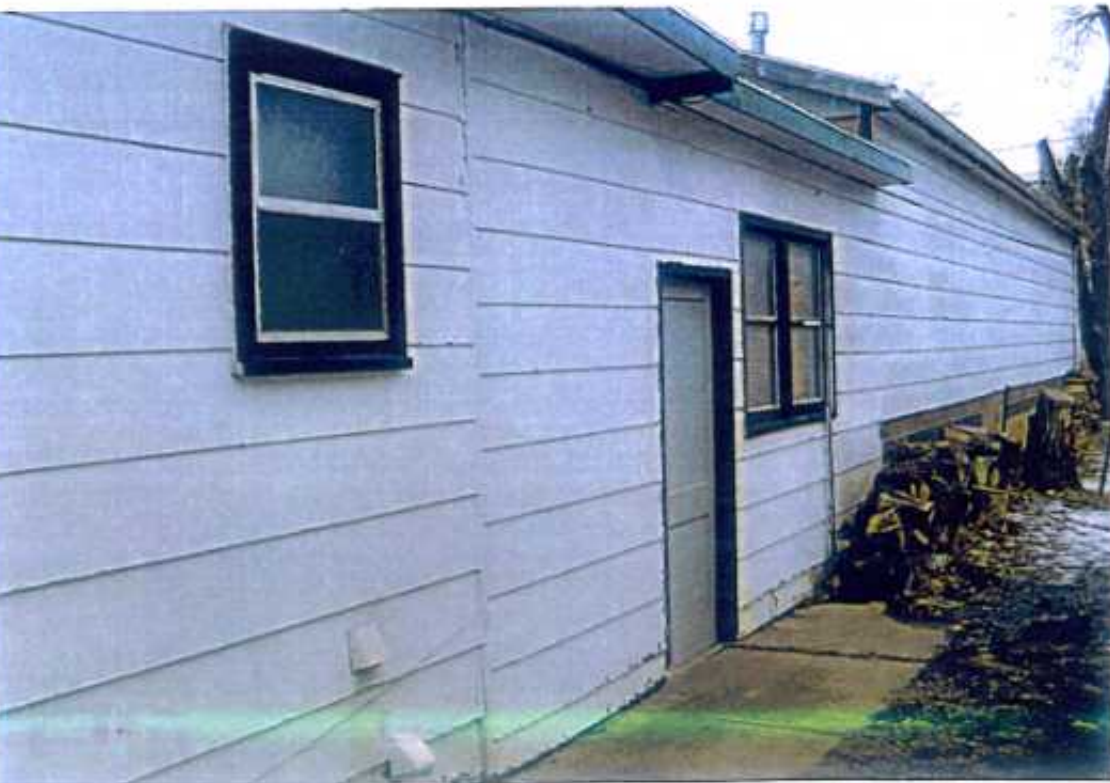
NORTH SIDE OF HOUSE
