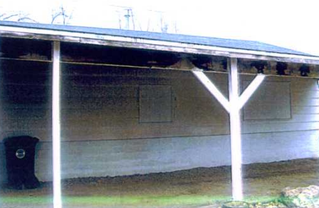
SOUTH SIDE OF GARAGE AND PORCH
