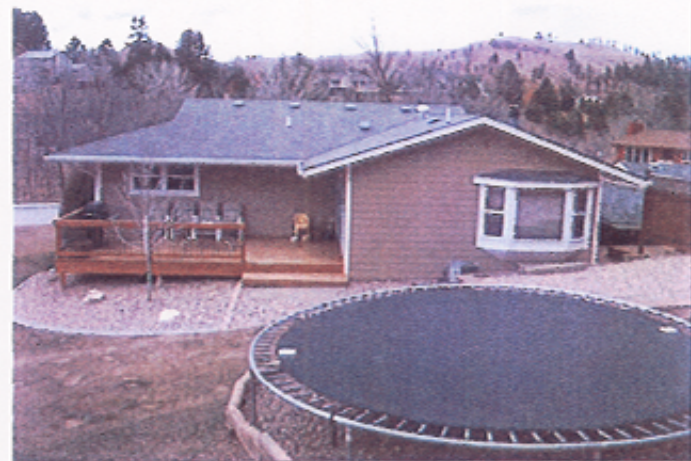
EXISTING DIGITAL PICTURE (REAR ELEVATION)
