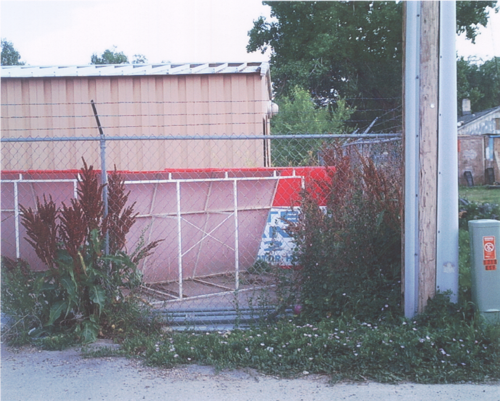
NORTH SIDE OF EXISTING STORAGE SHED
