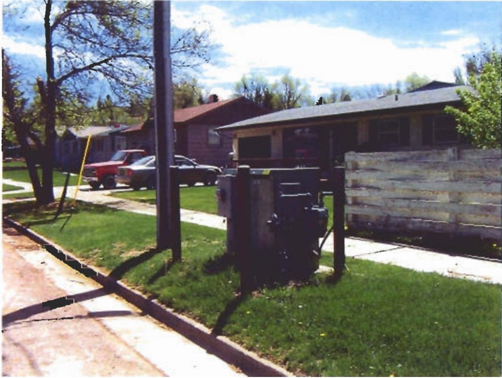
Located at 2733 West St. Patrick. Structure is 4' high, 1 1/2' deep and 3 1/2' wide.
