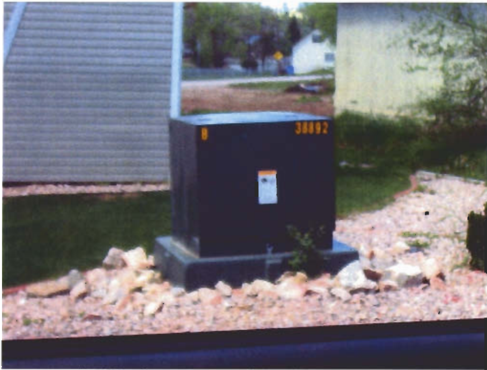
Outside of Apartments on the northeast part of town.
