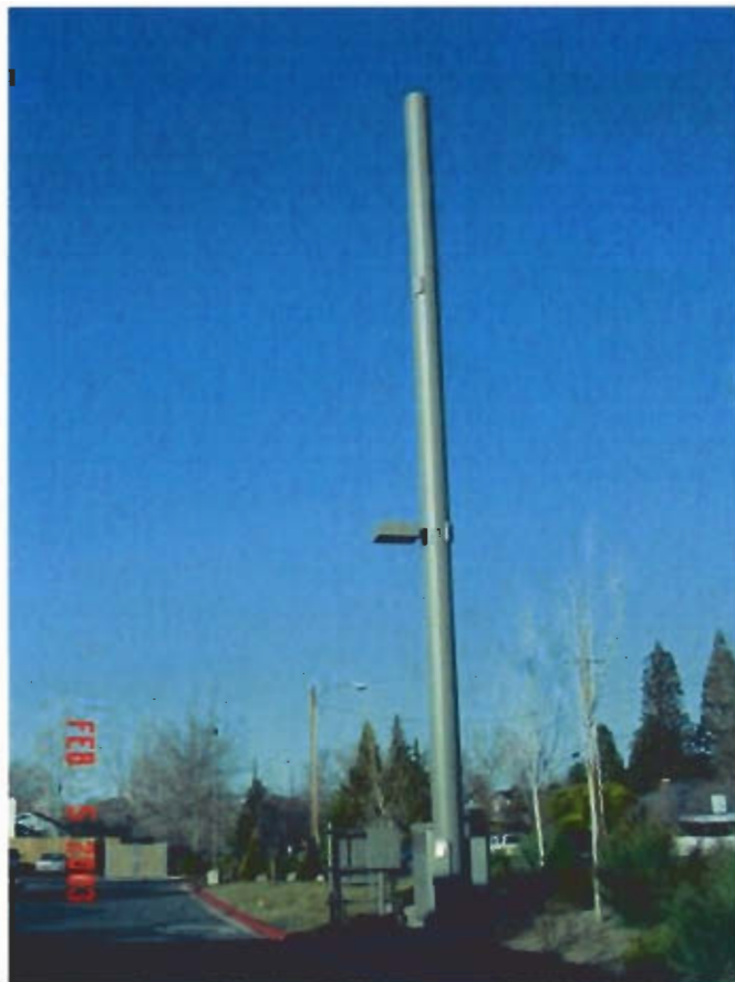
Modified Lightpole Installation in Reno, NV Residential Neighborhood
