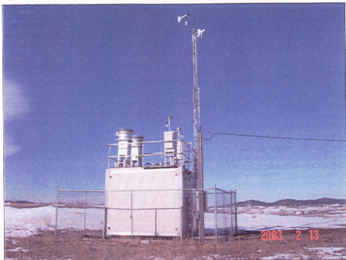
Example photos of a temporary air monitoring site with a mobile shelter.
