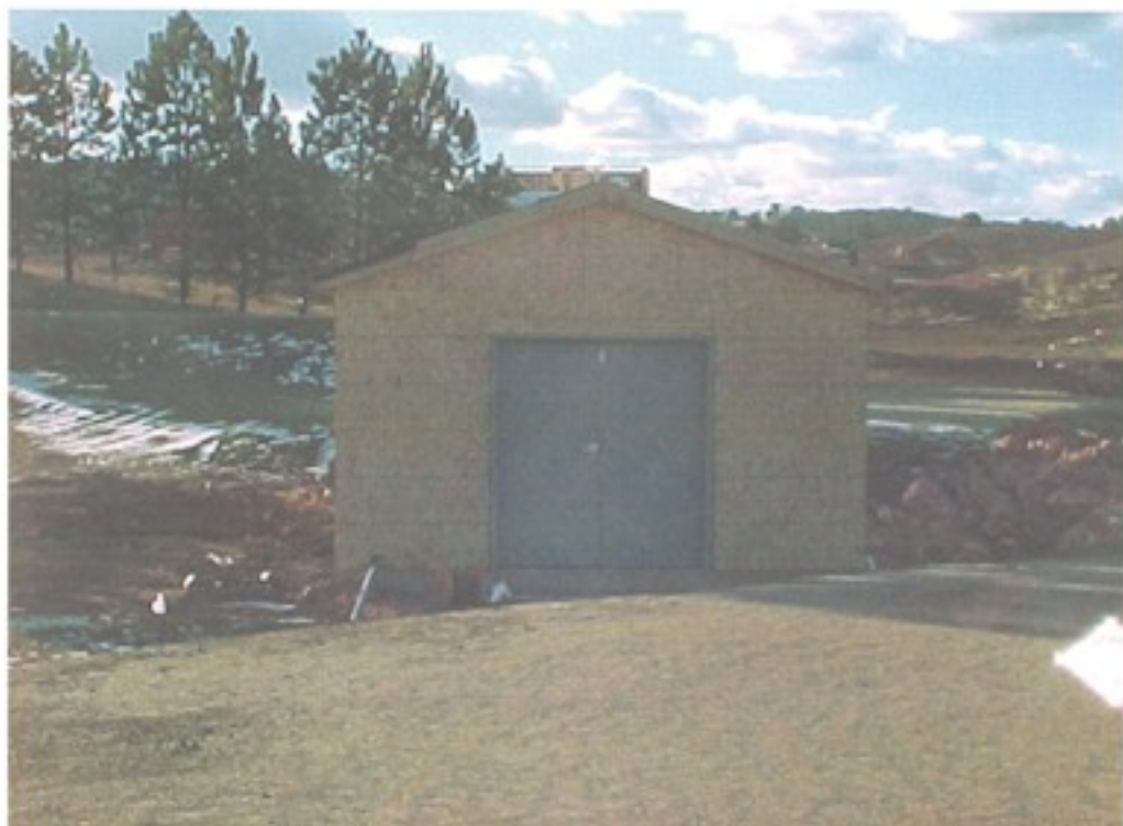
RED ROCK GOLF COURSE IRRIGATION PUMP HOUSE "EAST ELEVATION"
