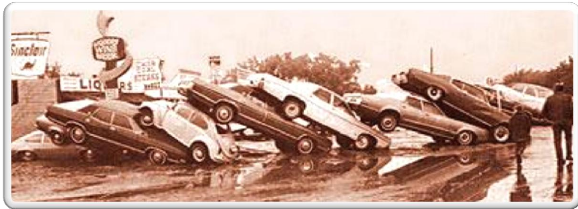
Aftermath of Rapid City Flood, 1972. Deaths - 238, Injured - 3,057, and 118 hospitalized
