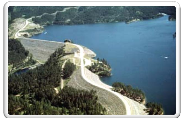
Pactola Reservoir and Dam on Rapid Creek, 34 miles upstream from Rapid City.
