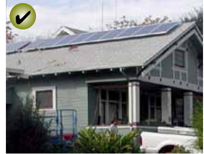
The addition of features such as solar panels should not interrupt the plane of the historic roof, and should be located below the ridgeline.
