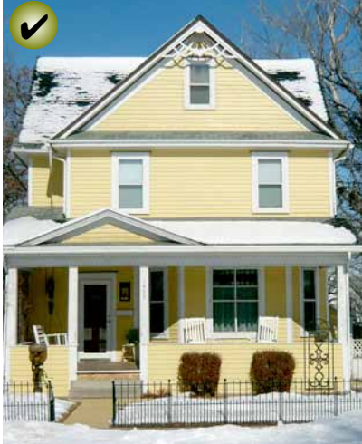
Preserve the original roof form of a historic structure.
