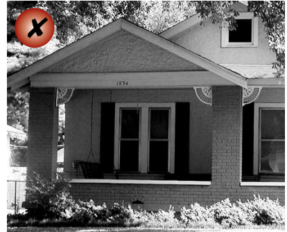
Avoid adding details that were not part of the original building. (These jig-saw details are out of character for a bungalow house.)
