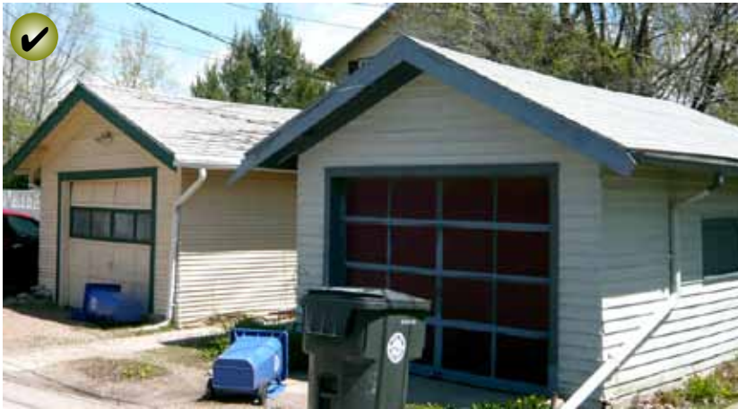
Preserve an existing secondary structure when feasible.
