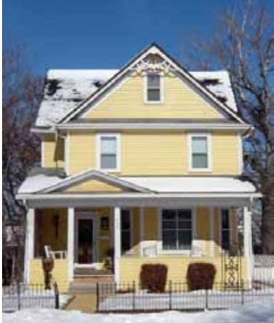
A “contributing building” in the West Boulevard Historic District
