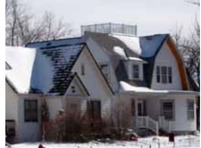
“Contributing buildings” in the West Boulevard Historic District
