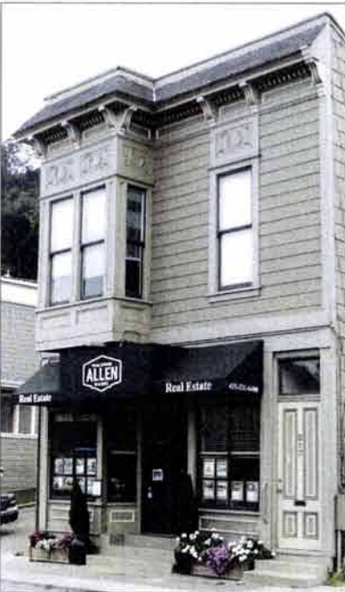
Compatible interpretations of traditional storefront components are appropriate where the original is missing.
