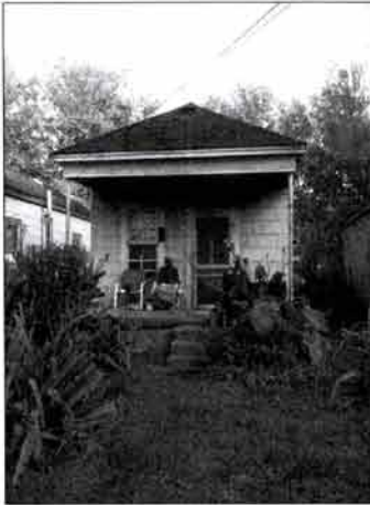
Many of the structures throughout the neighborhood are simple, two-room "shotgun" residences.
