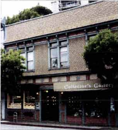
Preserve key features of a commercial storefront.
