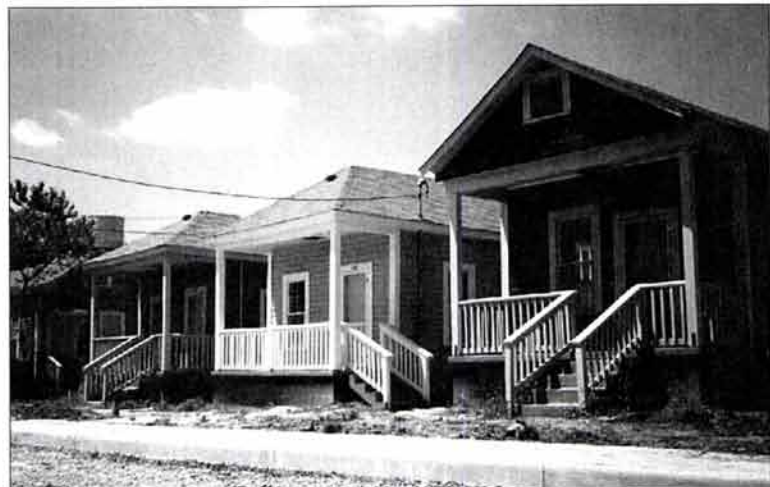
This recently renovated row of shotgun houses helps preserve the area's historical importance.
