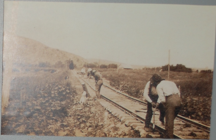
Construction 3 miles west of Rapid City looking west in 1880s
