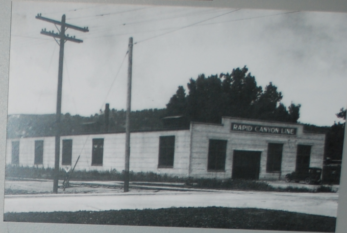
Rapid Canyon Line Rapid Canyon 400 West Broadway
