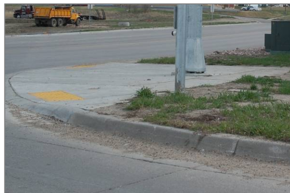
Figure 7. ADA-compliant curb ramp with tactile domes.
