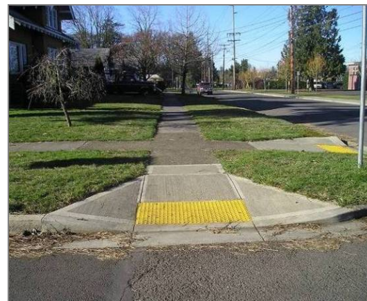
Example of an ADA-compliant perpendicular curb ramp
