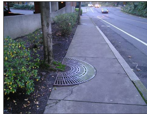
Tree well grates can create uneven sidewalk conditions and should not be placed within the thru-pedestrian zone.
