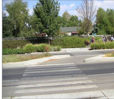
An offset crossing forces pedestrians to turn and face the traffic they are about to cross.
