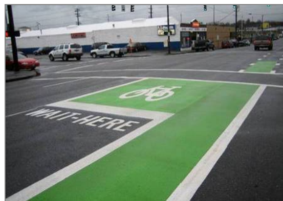
Bike boxes have been installed at several intersections in Portland, OR where right-turning motorists conflict with through bicyclists
