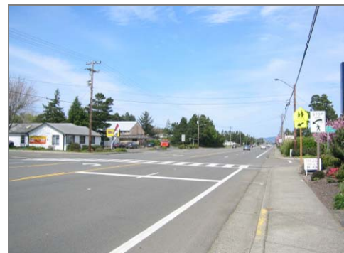
Advance stop bars alert motorists of pedestrians.
