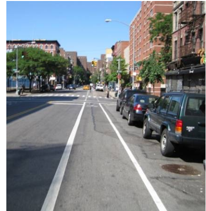
Bike lanes provide a travel lane for bicyclists that is separated from motor vehicle travel and parking lanes.
