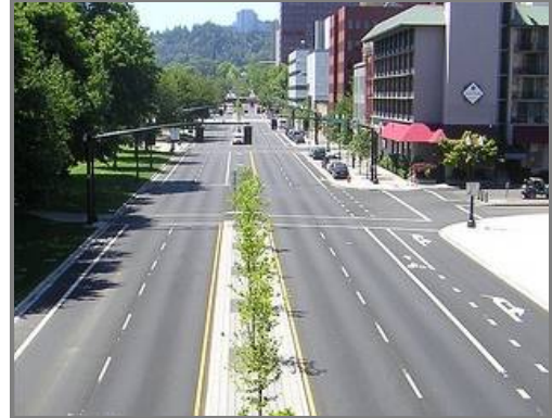
This street previously had 13' lanes, which were narrowed to accommodate bike lanes without removing a lane.
