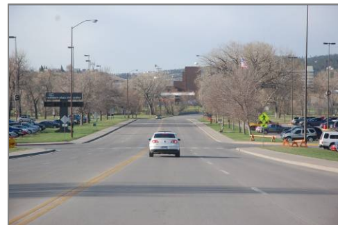
Figure 39. The crosswalk at Rapid City Central High School includes warning signage.
