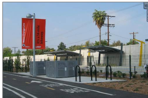
Figure 44. Rail-with-trail along Metro Orange Line, Los Angeles, CA.
