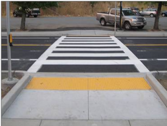
Figure 36. High-visibility crosswalk near a school in Fairfax, CA
