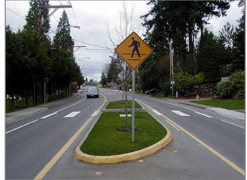
Figure 38. Pedestrian refuge island at mid-block crossing.
