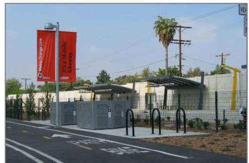
Figure 40. Rail-with-trail along Metro Orange Line, Los Angeles, CA.
