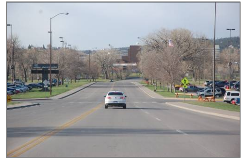
Figure 35. The crosswalk at Rapid City Central High School includes warning signage.
