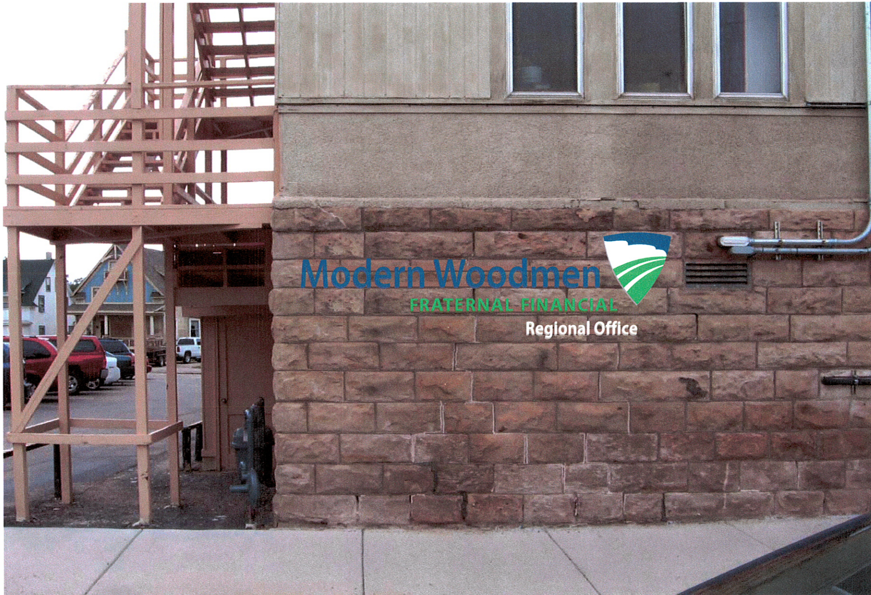
Routed 1/2" medex letters: 26" x 10', "M" = 8 3/4" tall, "F" = 4" tall, "R" = 4" tall, 1 1/2" rails painted to match brick
