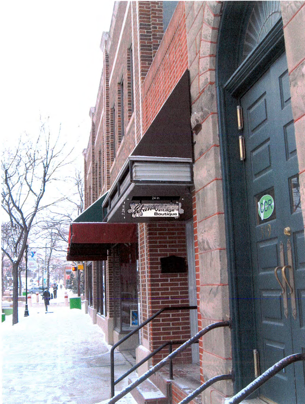
Double faced MDO pedestrian sign with graphics as per approved artwork. Sign to be suspended from under awning with steel structure.
