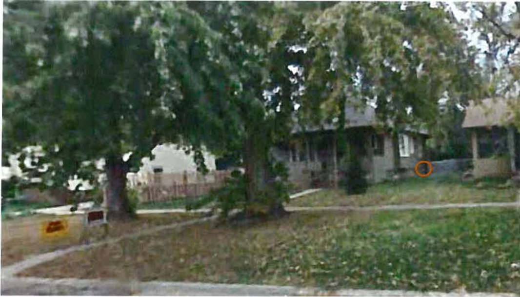
Back basement window to be replaced on north side
