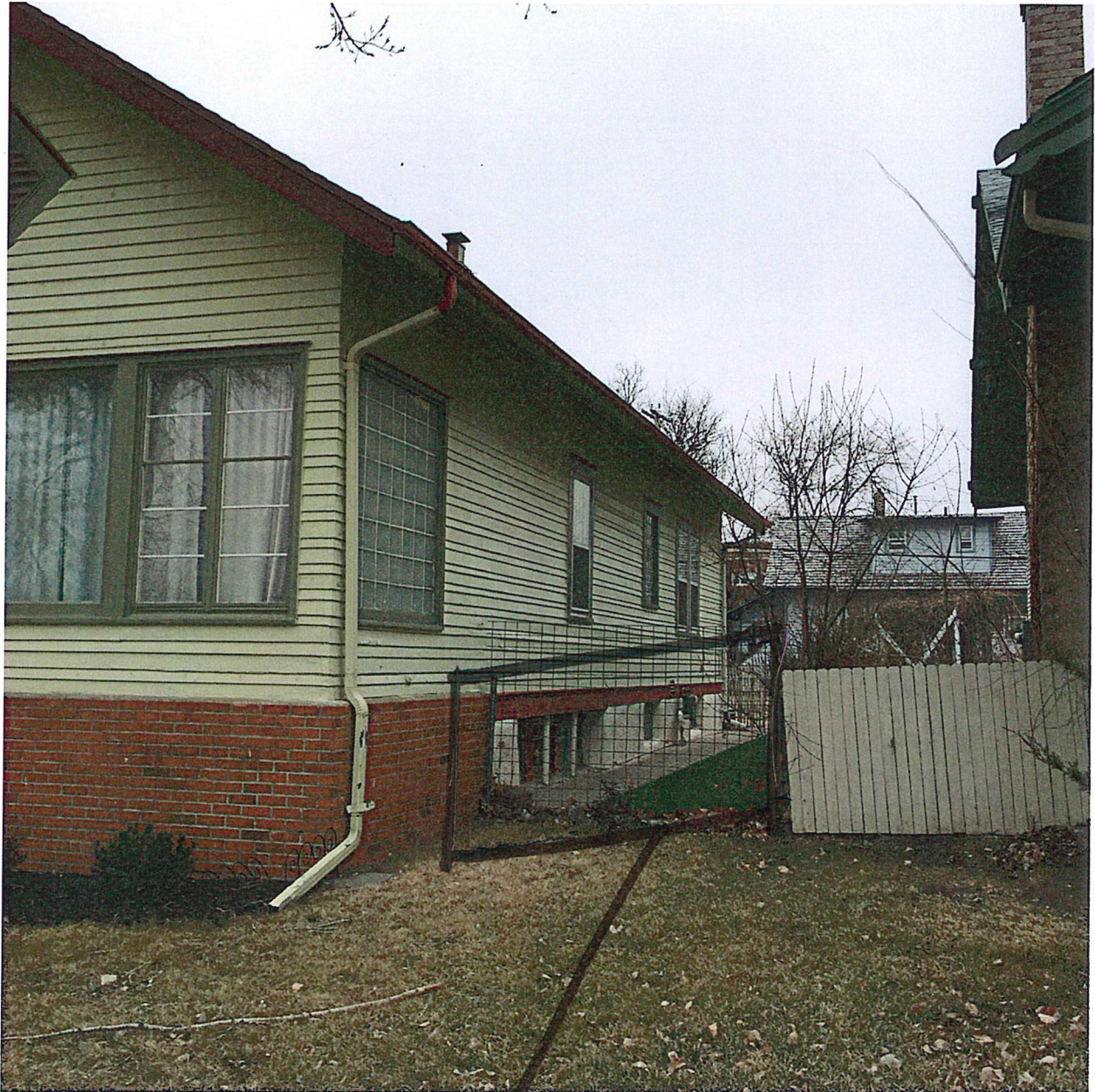
Street View of House – View of Impacted Area
