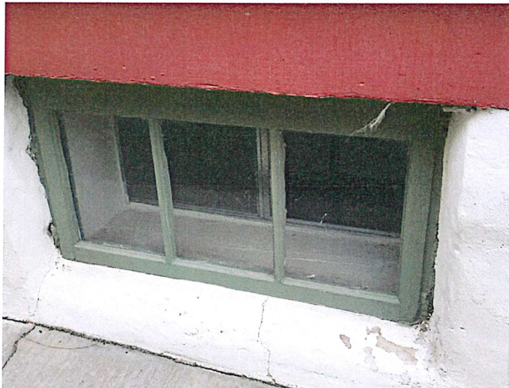
Window #1 – Exterior View
