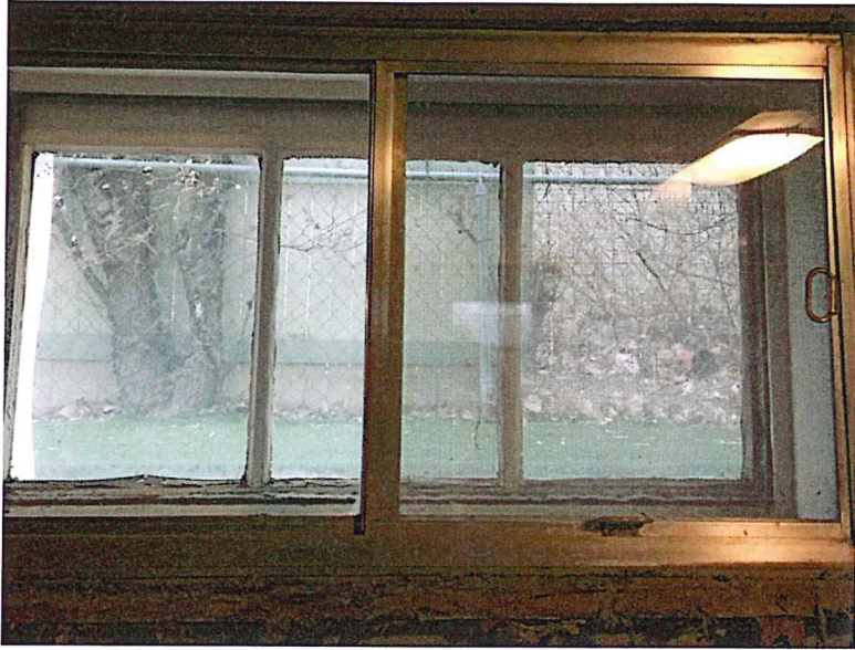
Window #2 – Interior View
