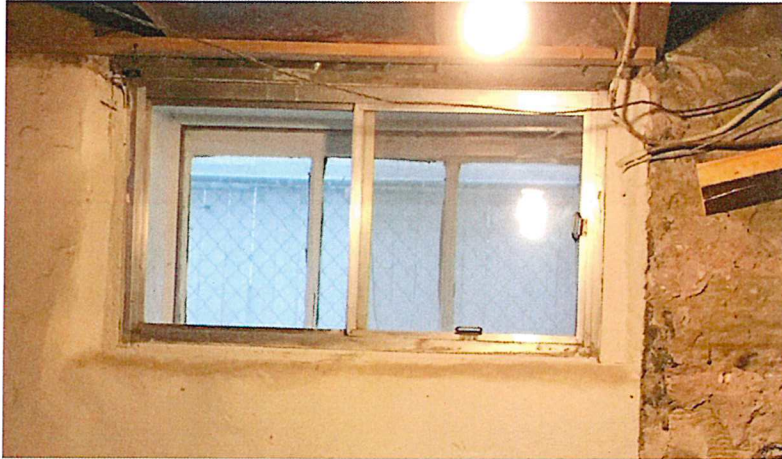
Window #1 – Interior View
