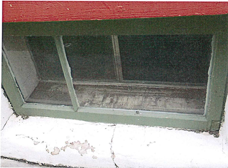
Window #2 – Exterior View
