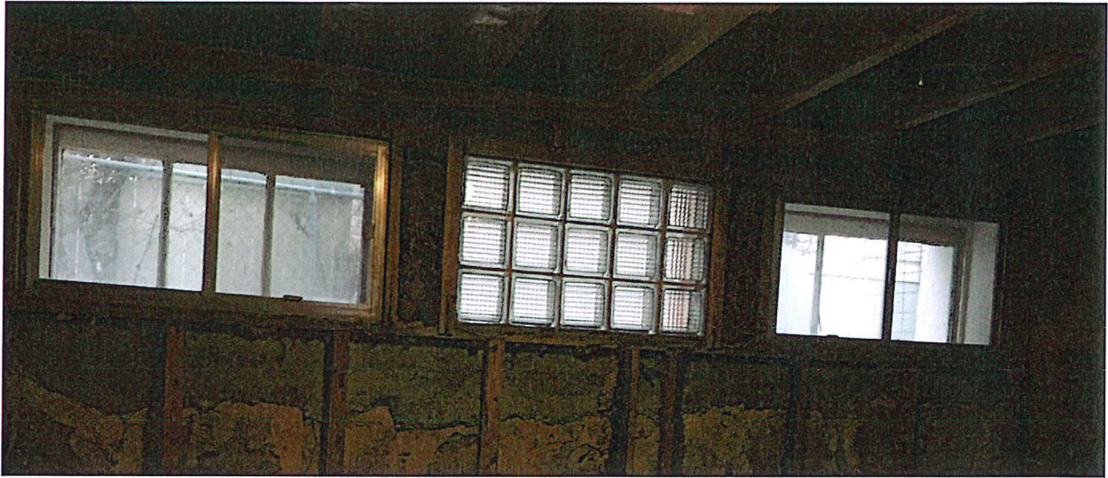
Windows #3-5 – Interior View
