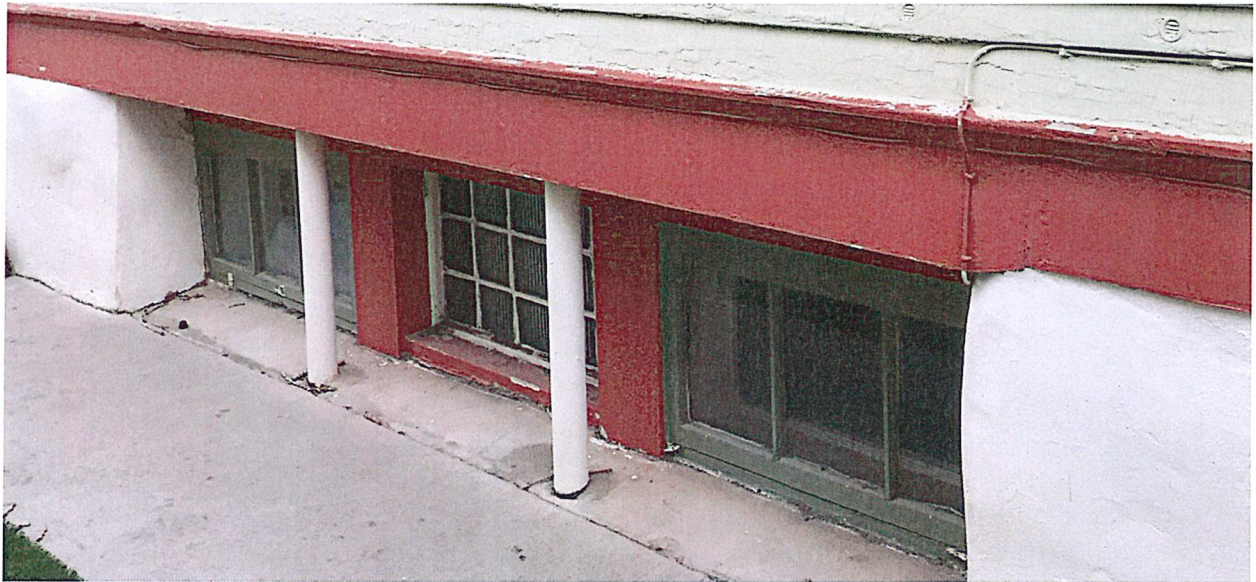
Windows #3-5 – Exterior View
