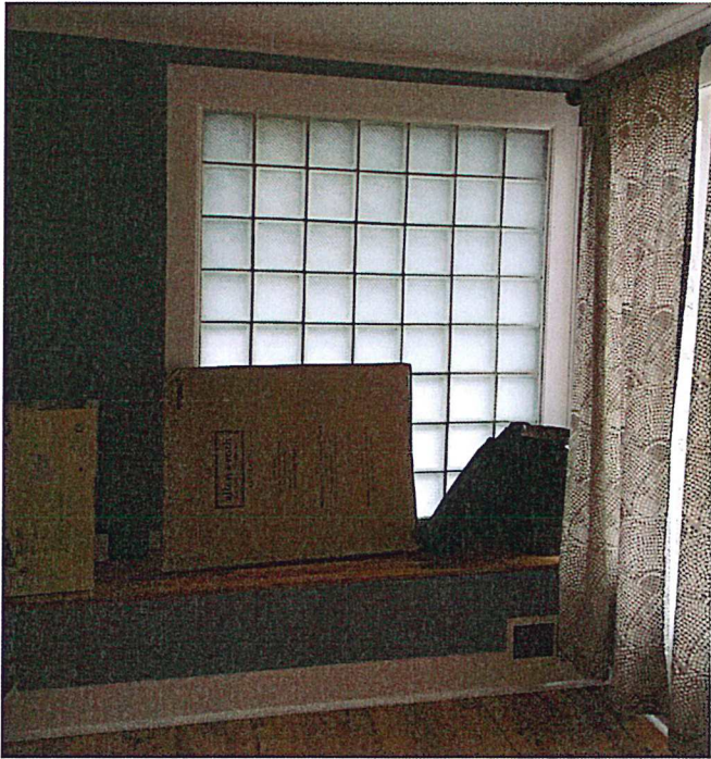
Existing Front Room Window
