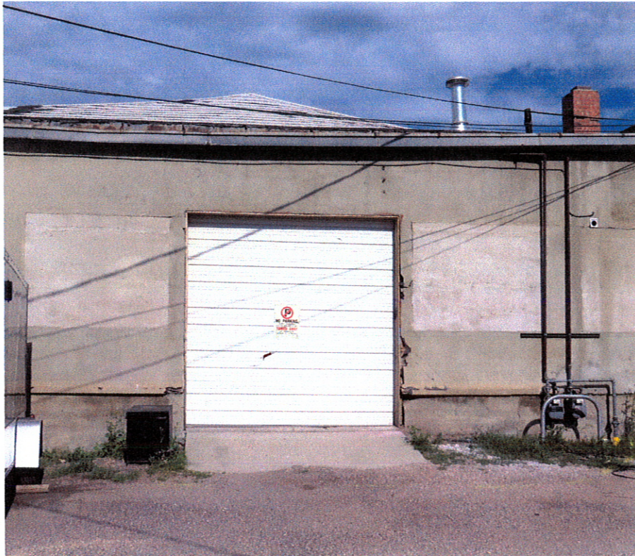
existing modern fiberglass overhead door 10' x 10'
